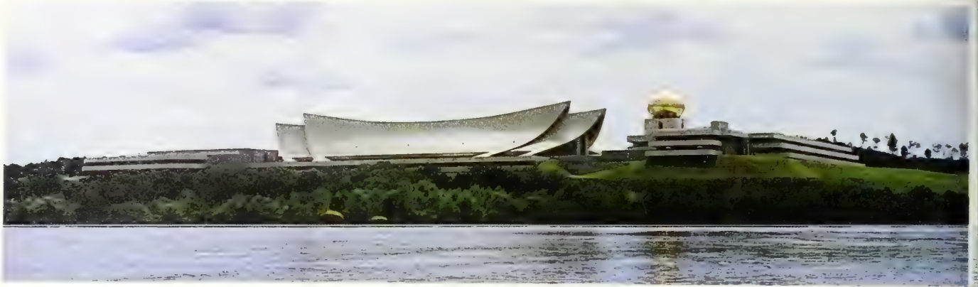
The dramatic Throne Building of the new Royal Palace of Brunei is a much-magnified modern version of the traditional longhouses of Borneo
