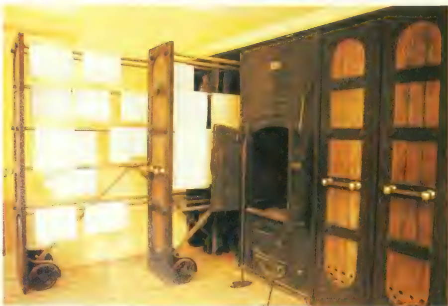
Top Kitchen at Manderston in Berwickshire (1901-05). Above Drying room at Hill of Travit, Fife, a chamber with a central stove to heat the air; "drying horses"—rails laden with clothes—were pushed in, pulled out.
