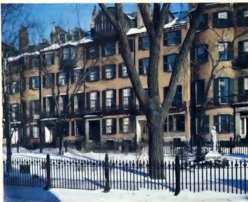
Louisburg Square's iron gate was installed in 1845, its statues seven years later
