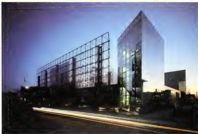
Indiana Bell Telephone Company Switching Center by Caudill Rowlett Scott, 1978, projects a bold High Tech profile.
