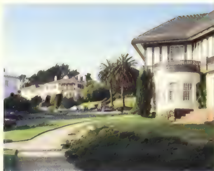
Presidio Terrace, shown at top in the original offering brochure, was carved out of the last vacant land near downtown San Francisco in 1905.
