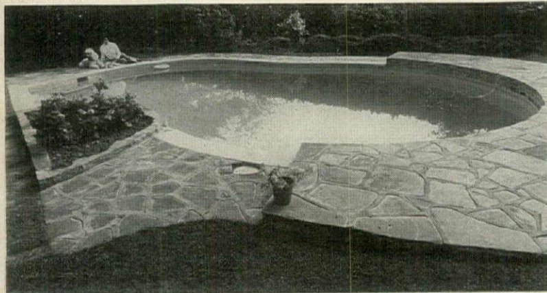
Pool with Gunite concrete shell, built by Classic Swimming Pools Ltd, who specialize in building individually designed concrete pools. Prices range from £2,000 upwards, but owners can keep costs down by organizing the site excavation and finishing themselves. Inquiries to Classic Swimming Pools Ltd, 138a London Road, Kingston-upon-Thames, Surrey.
