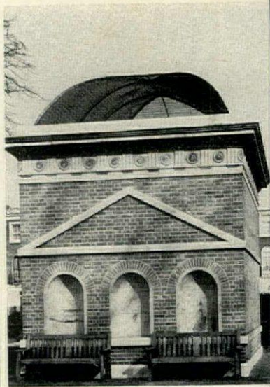
London Transport air vent in Gibson Square, Islington. See PYRRHIC PILE
