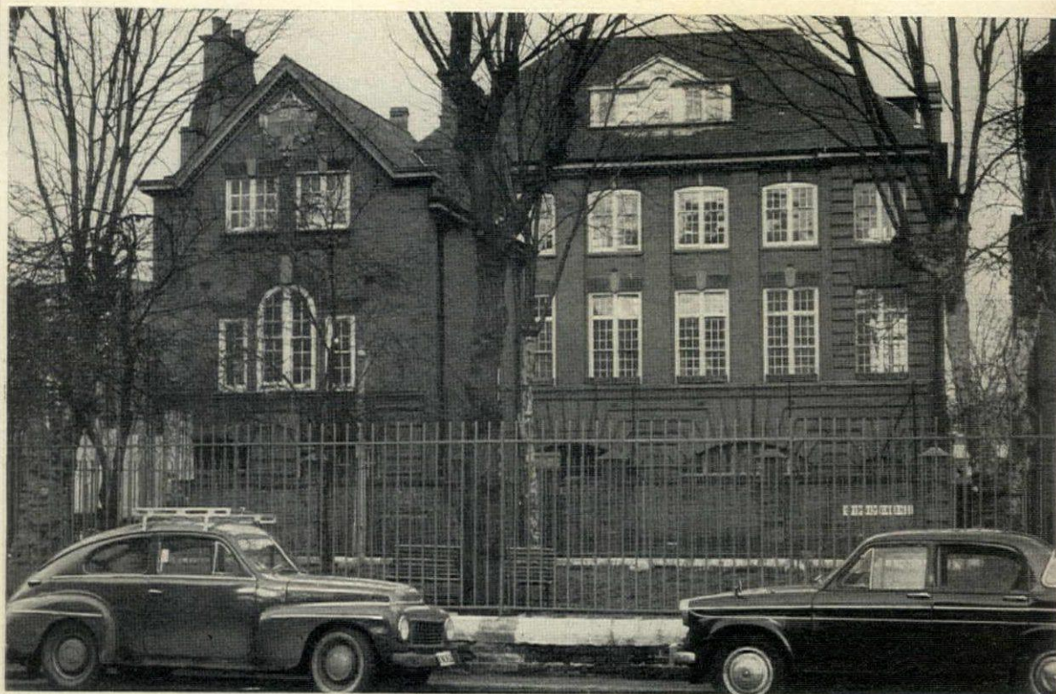
The exterior of the studios at Stepney Green in London's East End, made available by Space. (See this page)
