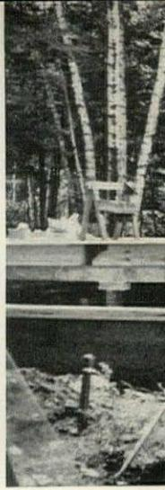
**ALEXIS PREPARES FOUNDATION FRAMING** for an ingenious, economical type of foundation he invented, which used two-thirds less concrete than a poured slab base. "It's a perimeter grade beam of poured steel reinforced concrete," he explains, "with a bed of crushed stone below, and a series of concrete piers or 'feet' 6 feet apart and extending 4 feet down."
