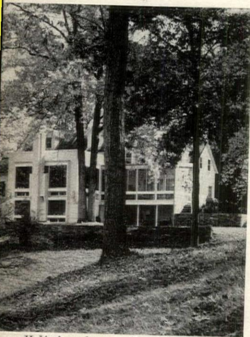
Half of porch was replaced by two-story addition, sheathed in clapboard to match rest of house. Stuccoed chimney outside end wall stands completely free from glass above top of upper fireplace. Inside the glass, shelf above floor level houses heating fins.
