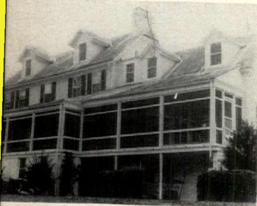
Before remodeling, a screened porch ran across entire back of the house at main floor level behind hall and living room.
