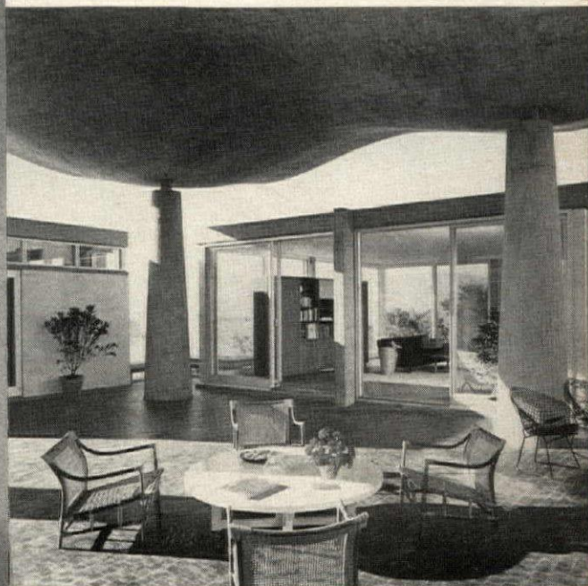
Almost Egyptian in style, the tapered columns supporting the canopy roof are of heavily textured concrete. Most of the furniture, inside and outdoors, was brought from Denmark.
