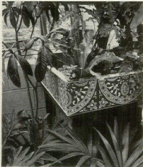
Floor tiles were cemented to bench sides, finished with aluminum strips. Tiles by Interpace.
