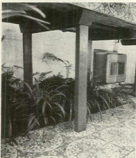
Ground beds under benches are filled with ferns and liriopis species. Heater is in wall at right.
