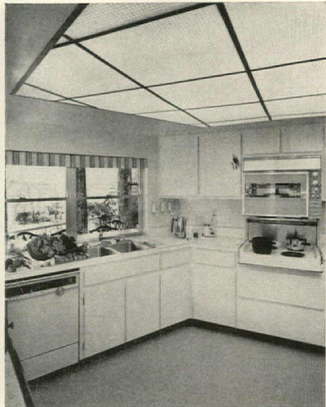
Kitchen has overhead fluorescents screened by a plastic grid.
