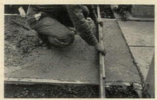
Make a concrete base 4 inches deep for the pebble finish (specify 5½- to 6-sack air-entrained concrete mix with maximum slump of 3 inches). Concrete should rest on a footing of tamped sand, gravel or crushed stone. For forms, use 2-by-4's. Level the surface of the concrete with a strikeboard.
