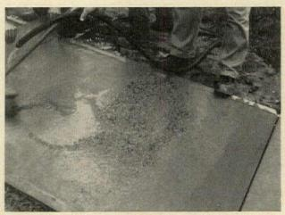
Expose the pebbles, after the surface is sufficiently firm, by removing the top coating of concrete with a medium stiff bristled brush. At the same time the surface should be hosed gently to wash away the coating dislodged by the brush. Care should be taken not to overexpose the pebbles. If it is necessary to move about on the surface, place boards, about 1 by  $1\frac{1}{2}$  feet, underfoot to distribute weight over a larger area.
