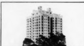
Dallas Park Hotel-Apartments
