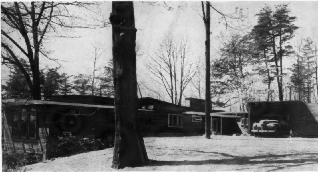
A shelf was cut into the hill to create a level motor court and one-story service wing. On the other side, the house has two floors built against the slope.
