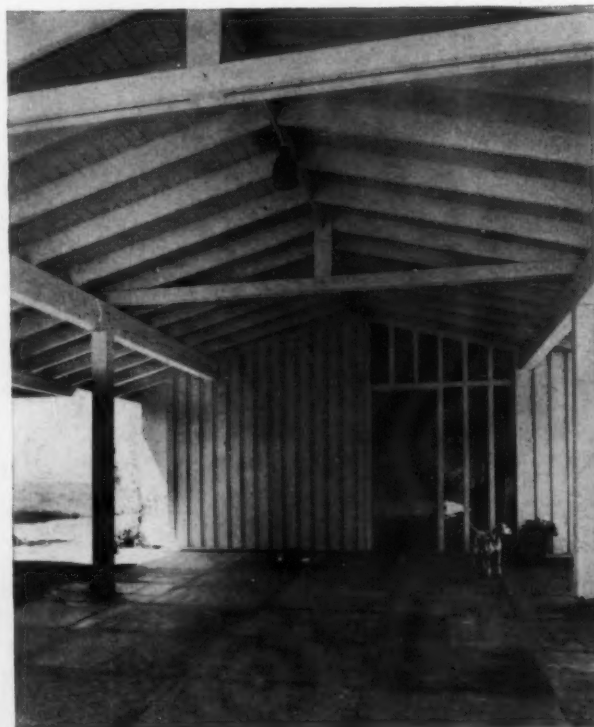
CHILDREN play on the front porch in rainy weather. Structural members form a frame for the glass in the wall of the entrance.
