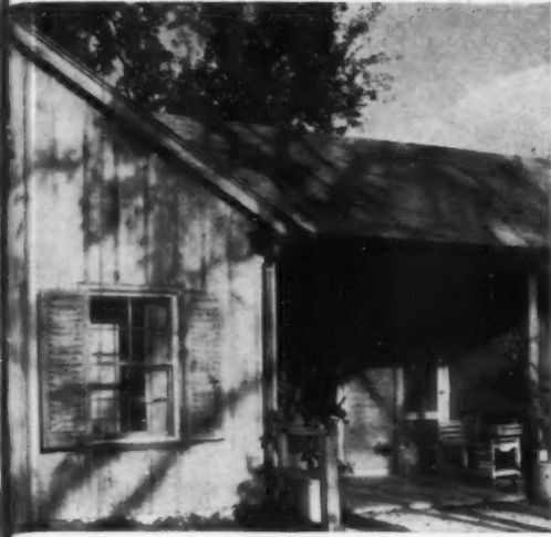
BOARD AND BATTEN—TRADITIONAL
