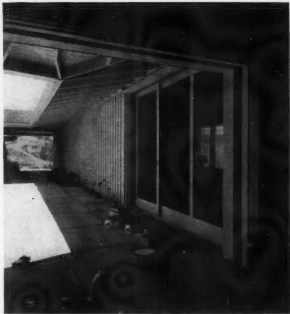
A WALL of the playroom facing the patio can be folded back. Rolling living room screens are shown in place.
