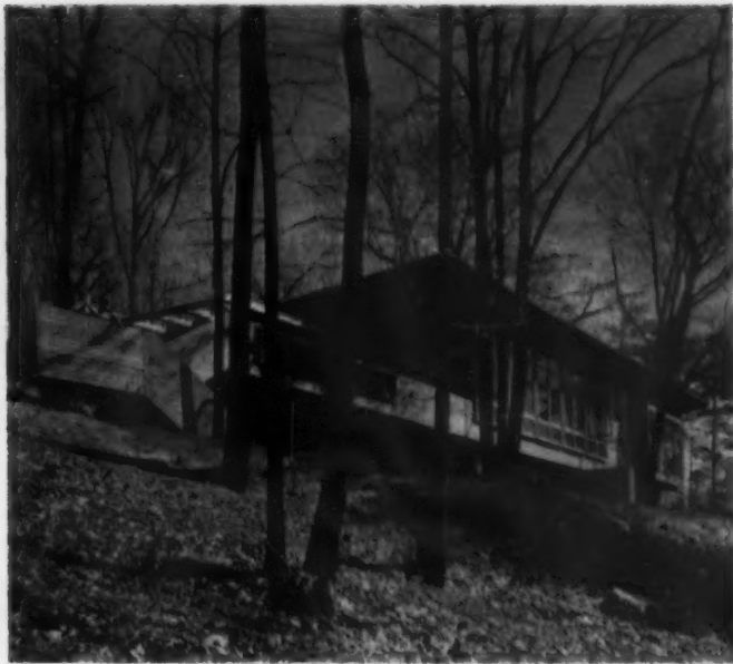
The house was cut into a sunny slope to protect it from cold northwest winds. The main rooms have window walls on the lee side.
