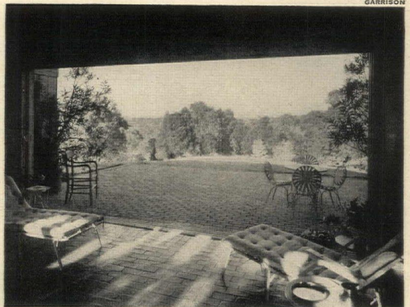
EAST TERRACE faces the edge of a bluff which slopes down to the lowland farms and the river. Sliding walls of the gallery (foreground) roll back on floor and ceiling tracks to admit breezes.
