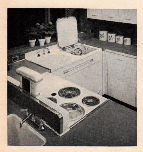
COOKING ACTIVITY CENTERS between sink and range; their relationship is the first consideration in any kitchen. In this plan, they are within arm's reach of each other, and are combined with broad work-tops, storage space for utensils and excellent lighting. The electric sink has a garbage disposal unit and an automatic dishwasher which will also wash pots and pans.
