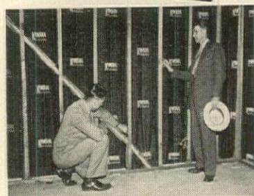
Mr. Steward Griffith and George Barbeau, contractors to whom Mr. Zehntbauer wrote, inspect a typical snug KIMSUL installation.
