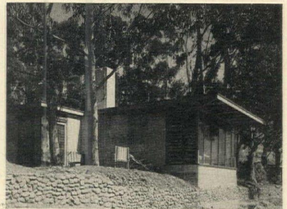
It is possible to get below the minimum 1000 square feet figure if family needs are simple enough. However, with no planned accommodations for children or guests, this design must be considered a special rather than typical solution.
