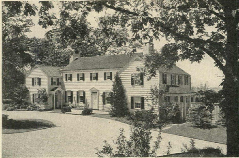
Carefully detailed windows are the very essence and spirit of traditional architecture. W. F. Dominick, architect; New York.
