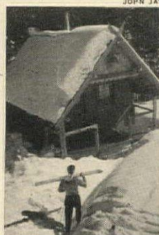
2. Arlberg's overflow house
