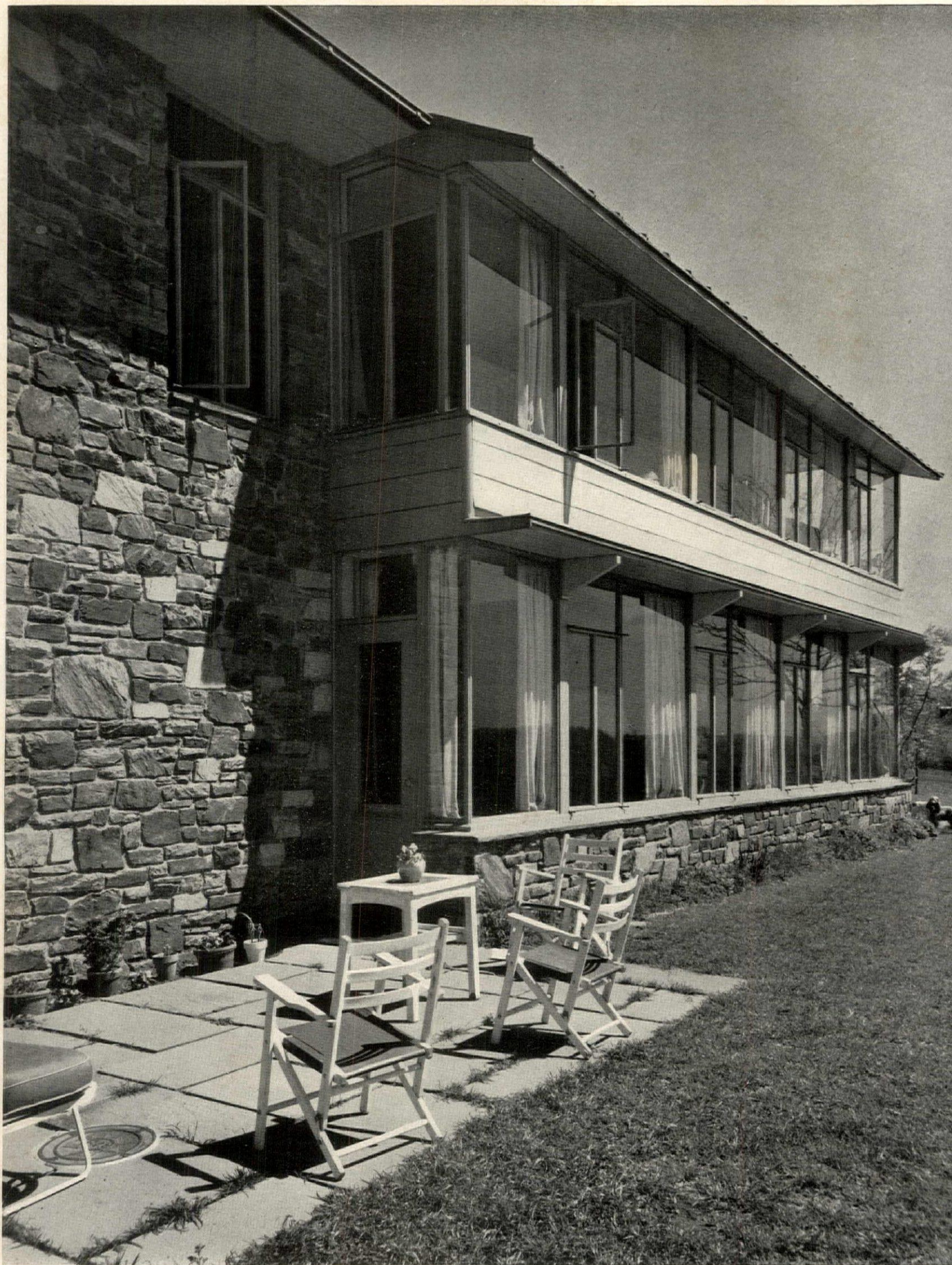
THE SOUTHERN FACADE of the Dechert house is designed to take advantage of the Winter sun
