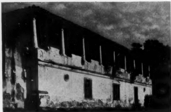
Roofed colonnades. Stucco-covered pillars support this roof in the old Fazenda Colubandé (above) near Niteroi. In the new seaplane station at Rio de Janeiro (right), by A. C. Lima, diagonal light steel tubes support the canopy.
