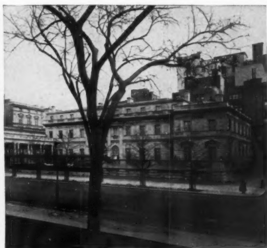
Now the Frick Museum, this building was sample of Sloane decoration in World War I, when it was home of the late great magnate. To same era belongs job for Charles M. Schwab.
