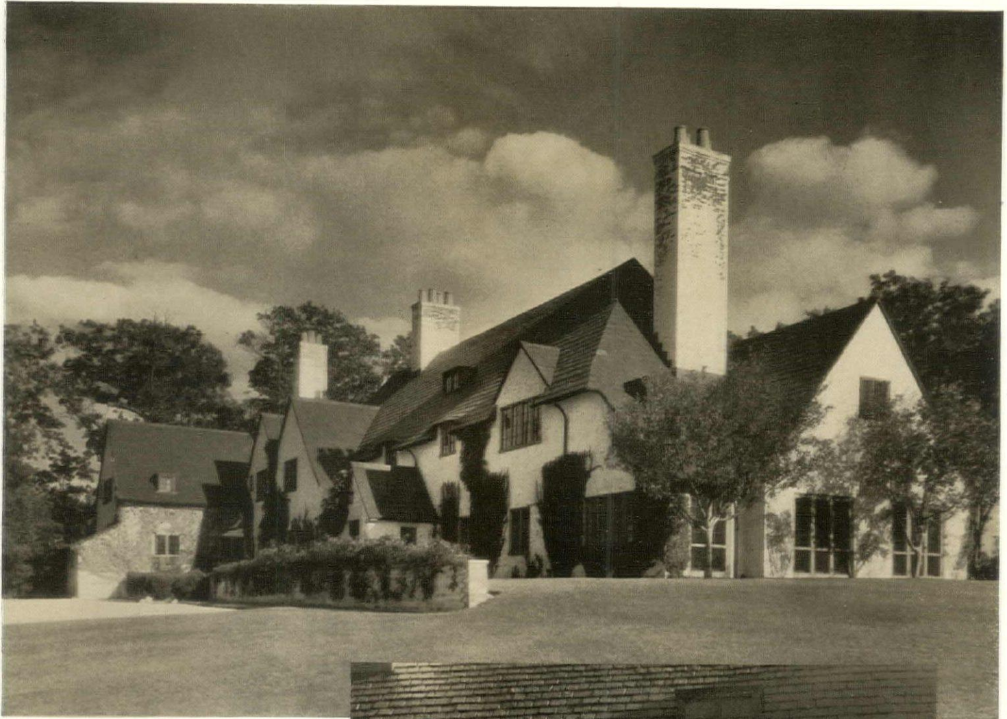
ENTRANCE APPROACH AND NORTH FAÇADE
