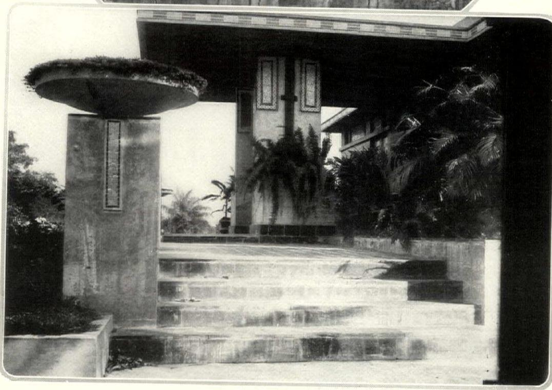
Monolithic concrete construction makes the house fireproof. The broad overhanging slabs that shadow the porch were cast in one piece. So were the decorative flower vases
