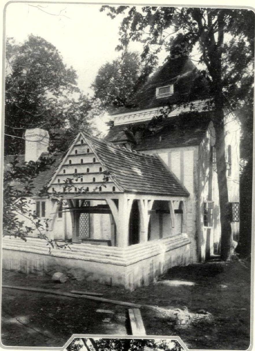
(Below) A wall constructed of brick and half-timber showing the manner in which brick is laid up between the timbers. Clinker brick fitted together in an irregular fashion is used. The mortar joints are left unraked
