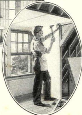
Anyone who can use a saw and hammer can finish off an attic room with Celotex. You simply nail the broad, light boards to the studding and rafters. Celotex not only shuts out heat and cold but converts your old attic into an attractive, livable room.
