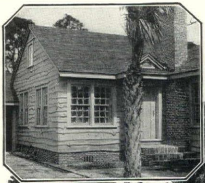
WEATHERBEST semi-thatch Stained Shingle Roof in a selection of variegated colors of green, gray, brown and red. Most effective with foliage and over interesting sidewalls of long-leaf pine boards with rough edges. Arch't and owner, Roland A. Phillips, St. Petersburg, Fla.
