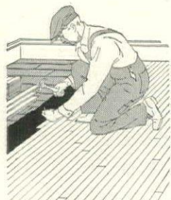
Remodel one room at a time, if more convenient. No woodwork need be disturbed, except the quarter-round at the baseboard.
