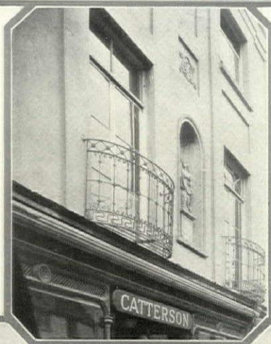
Wrought iron and straight narrow bands of iron bent to the desired shape are used in the individual window balconies shown at the left. Cast rosettes mark the crossings of the lattice which completes the top of both these graceful early 19th Century designs
