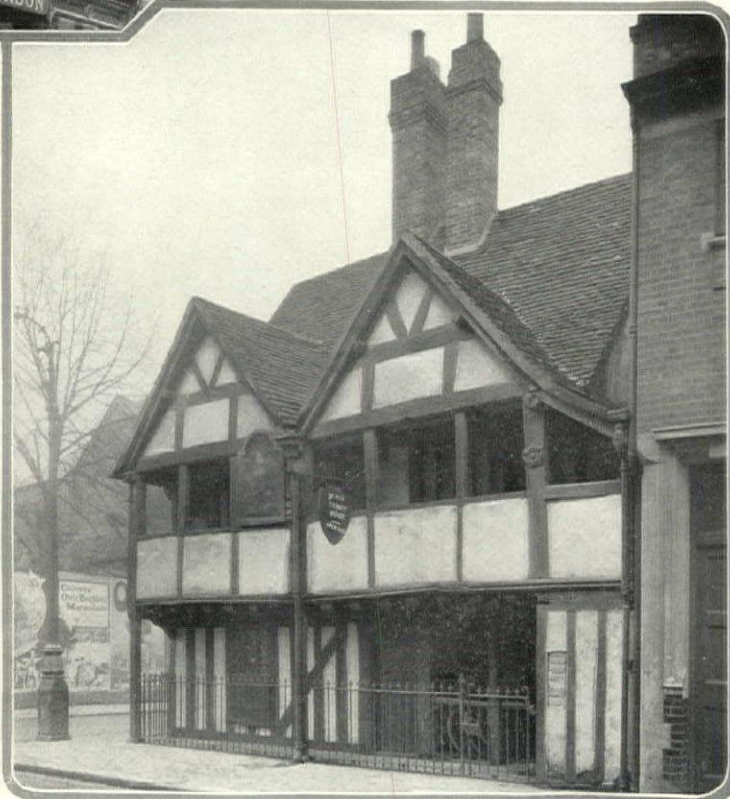
When correctly conceived the balcony can be a harmonious feature of the half-timber house. In the Elizabethan example below it is a spacious place of substantial construction and becomes an integral and valued structural part of the house design
