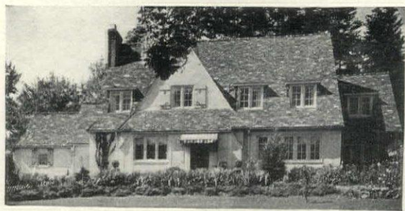
Blended roof shingles stained with Cabot's Creosote Stains Reed & Corlett, Architects, San Francisco
