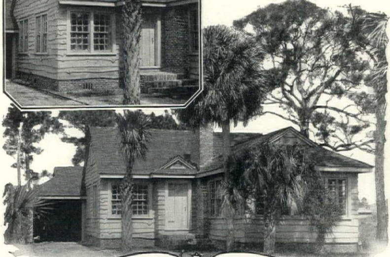
WEATHERBEST semi-thatch Stained Shingle Roof in a selection of variegated colors of green, gray, brown and red. Most effective with foliage and over interesting sidewalls of long-leaf pine boards with rough edges. Arch't and owner, Roland A. Phillips, St. Petersburg, Fla.
