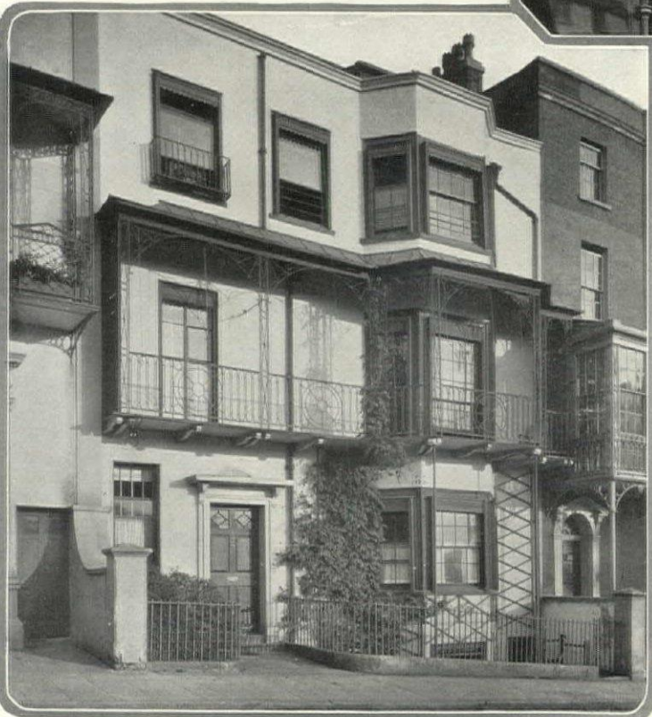
(Below) Here the balconies have been brought forward to follow the contour of the house front, but their roofs are high enough not to affect the light of the windows. They are of the early 19th Century and found on a house in Gloucester, England
