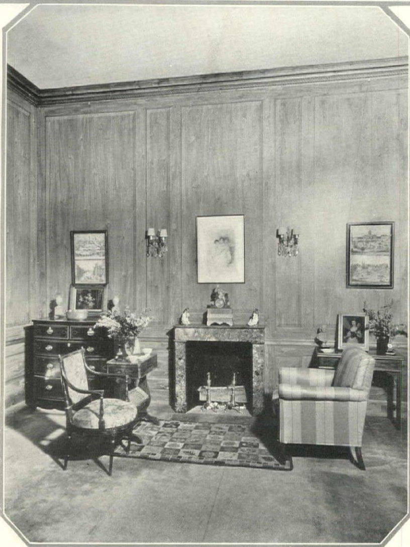
The Tudor background shown in the dining room above is in reality a plaster wall marked off in small squares with narrow wood moldings. The whole is then grained in oak to resemble old paneling
