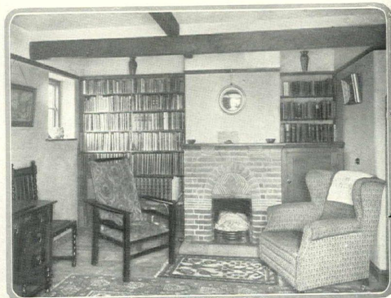
The living room has a big bay window facing south and a smaller one to the west. On either side of the brick fireplace are built-in bookshelves, and to the right a deep cupboard.
