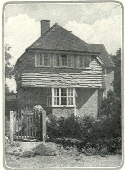
This cottage was designed by the architect, Edwin Gunn, to receive as much sunlight as possible. Elm weather-boarding gives the house a countrified appearance.
