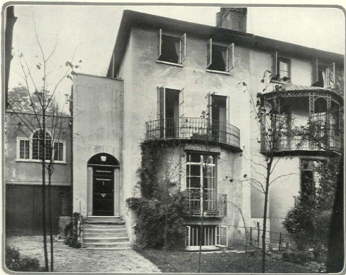
A London house carries two pleasing balconies of the early 19th Century. The open one at the left is made on the top of a semi-circular bay, where it adds marked lightness and grace. Its mate has been developed into a veranda with pagoda-like roof
