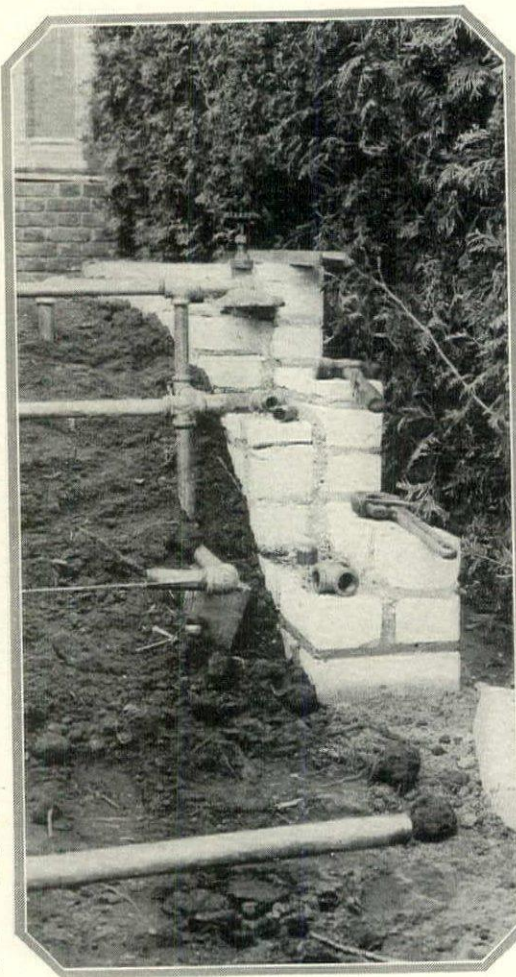
Transverse pipes serve as water distributors and supports for the sod. They should provide a riser height of 6" and a tread width of 16" to 24"
