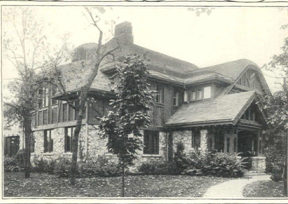
Residence of B. C. Keeler, Mason City, Iowa. Hollow Tile with combination stone and face brick exterior
