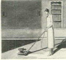
9. I attached the steel wire brush armed with a pad of steel wool and went over the prepared portion of the floor.
