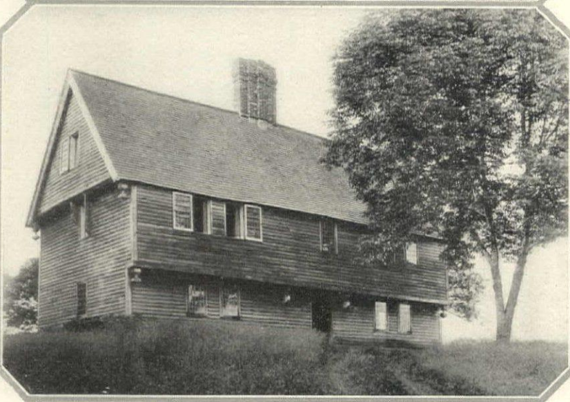
The local Historical Society of Topsfield found the Capen House in poor state — original clapboards and windows gone. It was bought and restored
