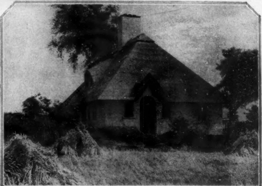
No other roofing material seems to have the fine flexibility of thatch, as in this delightful cottage by Basil Oliver
