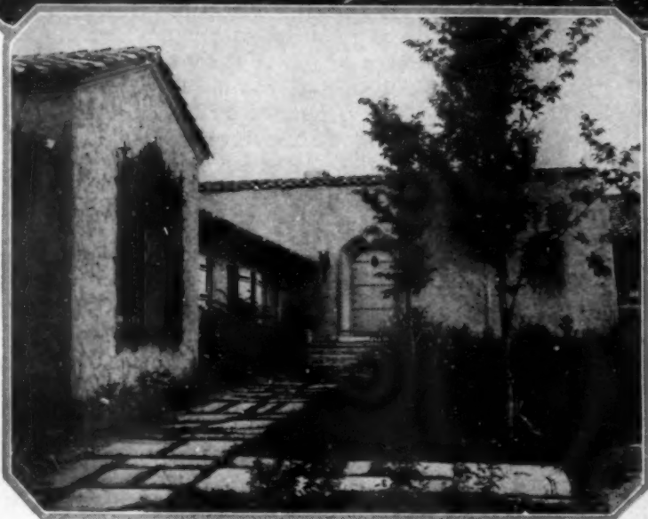
Carrying out the Spanish idea in its architecture, the house has stucco walls and a red tile roof. The sitting room window is enhanced by a decorative grille and the door into the arcade by a decorative frame in the Spanish style
