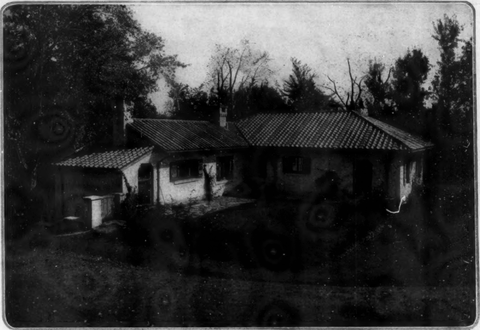
The building above is the gate lodge which stands at the estate entrance, some distance from the farm group. Its color and its architectural style, however, are similar to the other buildings
