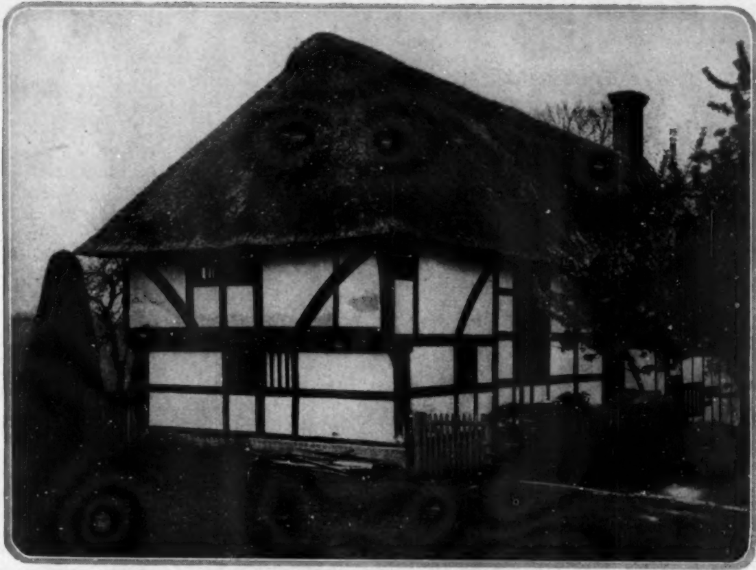
The thatching of this XVth century English cottage gives evidence of the extraordinary and unexpected durability of this sort of roofing
