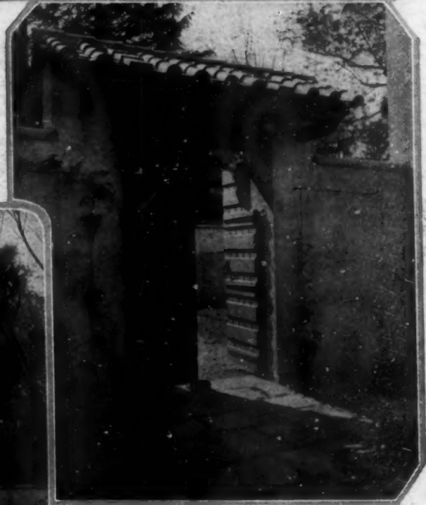
In the gardener's cottage, with its graceful double arch and splendid proportions, can be seen the effectiveness of the method used in laying the tiling. One row of flat tiles is laid between every four vertical rows of half-round tiles, giving an unusual texture to the roof
