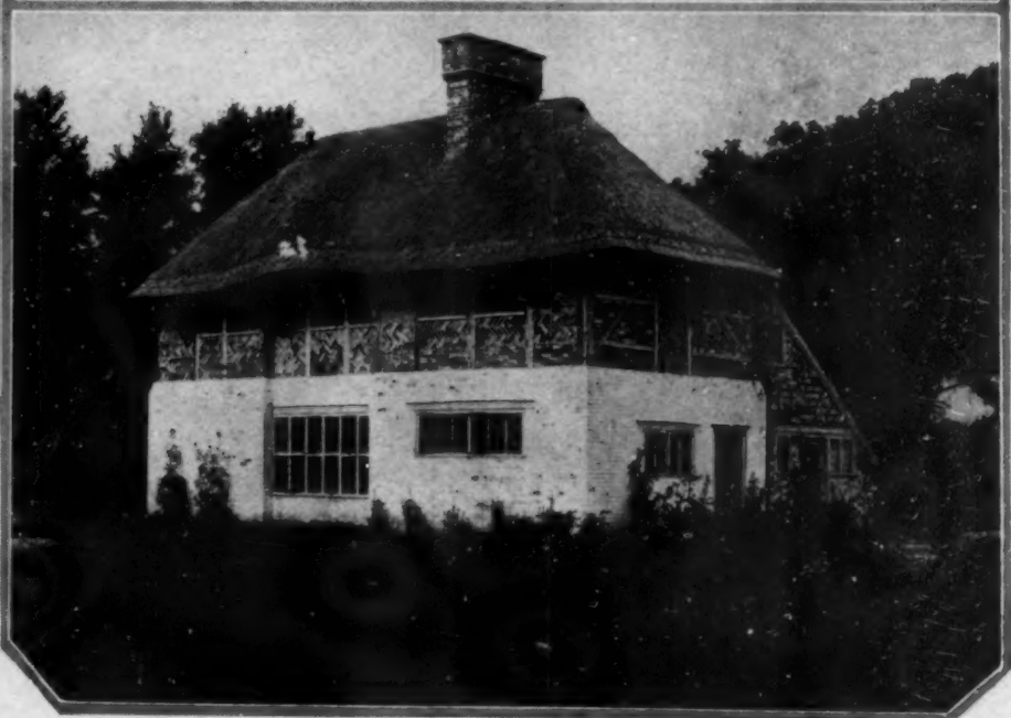
A modern English example of thatching shows how the material is held along the ridges and eaves by hazel "swais".
