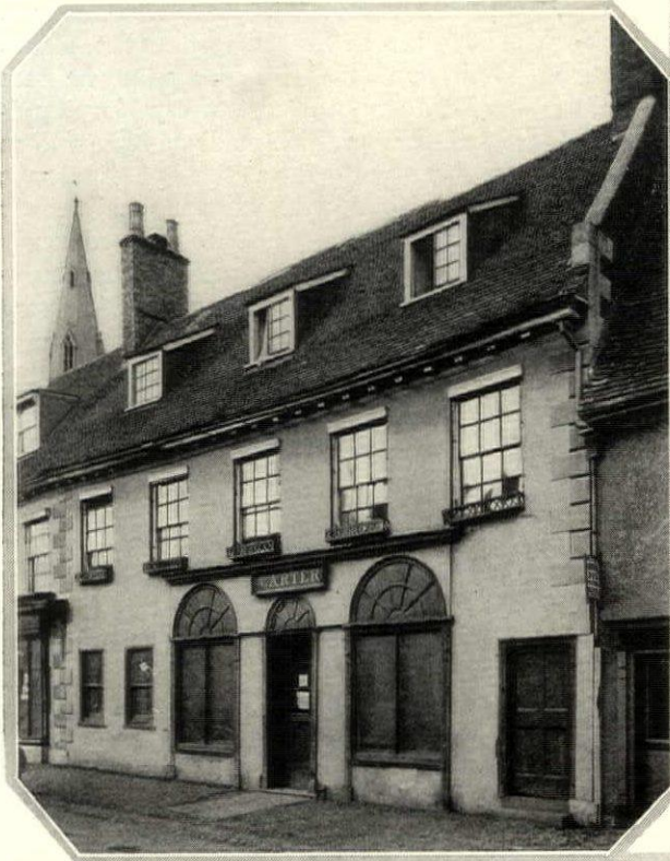
The unusual features of these dormers above a shop at Kimbolton, England, are their short, upward sloping roofs contrasting sharply with the pitch of the main roof, and the white large board at the top of the sides left showing to emphasize the presence of the dormer
