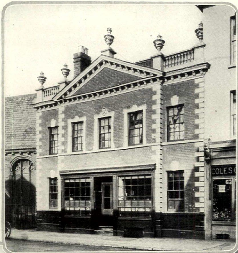
An old shop in Gloucester, England. The white quoins, in sharp contrast with the red brick, not only define the projection of the central bay, but, along with the white keystones, white architraves, white cornice and white balustrades, give liveliness to a really simple building
