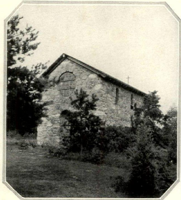
The west end of the chapel at Whitehall is broken by a circular window and the entrance door. The windows are located high in the walls and directly under the eaves
