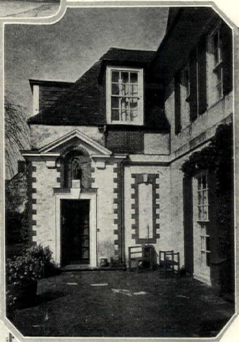
In this terrace front of an English country house by Sir Edwin Lutyens the red brick quoins serve an obvious decorative purpose. They emphasize the niche and blank wall
