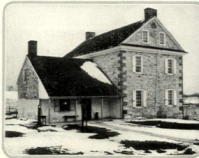
A farmhouse near Reading, Pa., in which the quoins, purely decorative, represent a structural style of the locality. They define the corners and lend the walls contrasting colors
