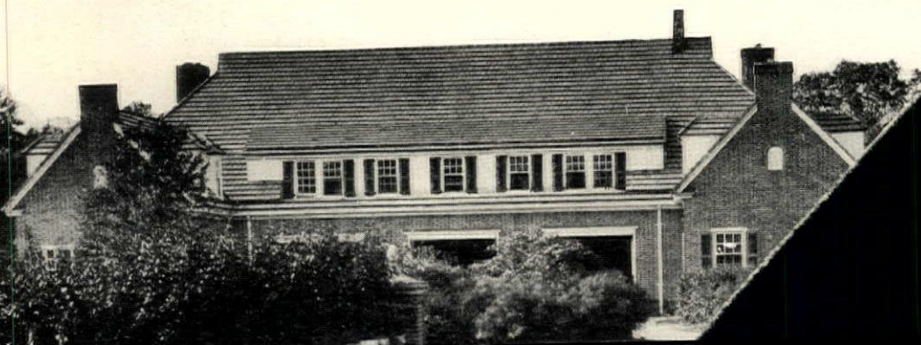
Garage and three housekeeping apartments
