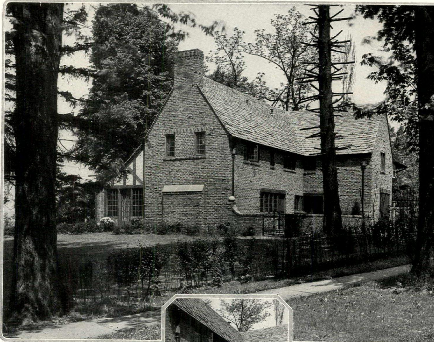
An interesting, but not too-artificial texture has been accomplished by the skillful use of clinker-faced brick. The owner is W. Jule Day, at Douglastown, L. I., and the architect is Frank J. Forster
