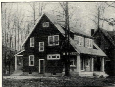
Residence of Walter M. Collins, Builder, Bayside, L. I. Insulated with Cabot's Quilt. Stained with Cabot's Creosote Stains
