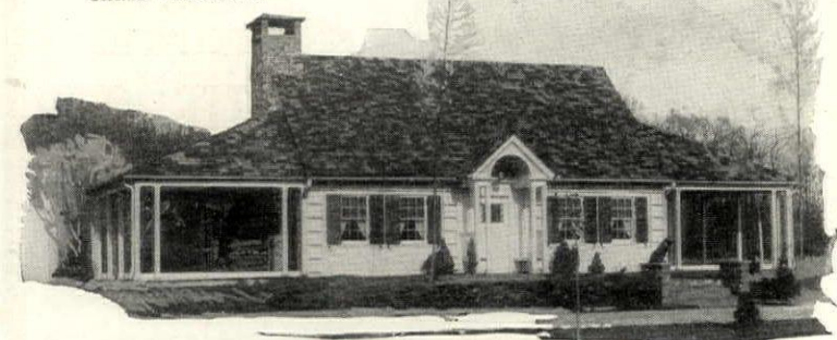
Arch. Miles B. De Chand, Reading, Pa., used "CREO-DIPT" Stained Shingles in variegated colors, on roof, and on side walls, 24-inch "CREO-DIPT" Stained Shingles with wide exposure in Dixie White for true Colonial white effect.
