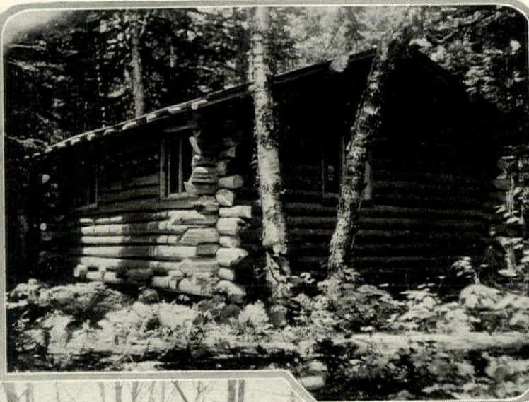
There should not be a too strict regularity in the length of the logs
