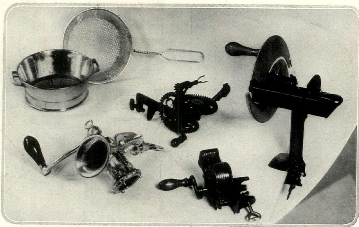
Among the many instruments that help take the drudgery out of summer canning are those which assist in the preparation of fruit and vegetables. Thus the meat grinder, a sine qua non in any self-respecting kitchen. Then, to the rear of this, a fruit parer; the fruit is spiked on the three prongs and a turn of the handle does the rest. At the front is a bean slicer and to the right a fruit slicer. A sieve and a culinary basket complete the picture
