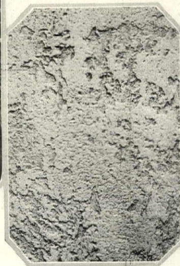
A detail of a new plaster wall finish which has been developed to produce varied combinations of texture and color
