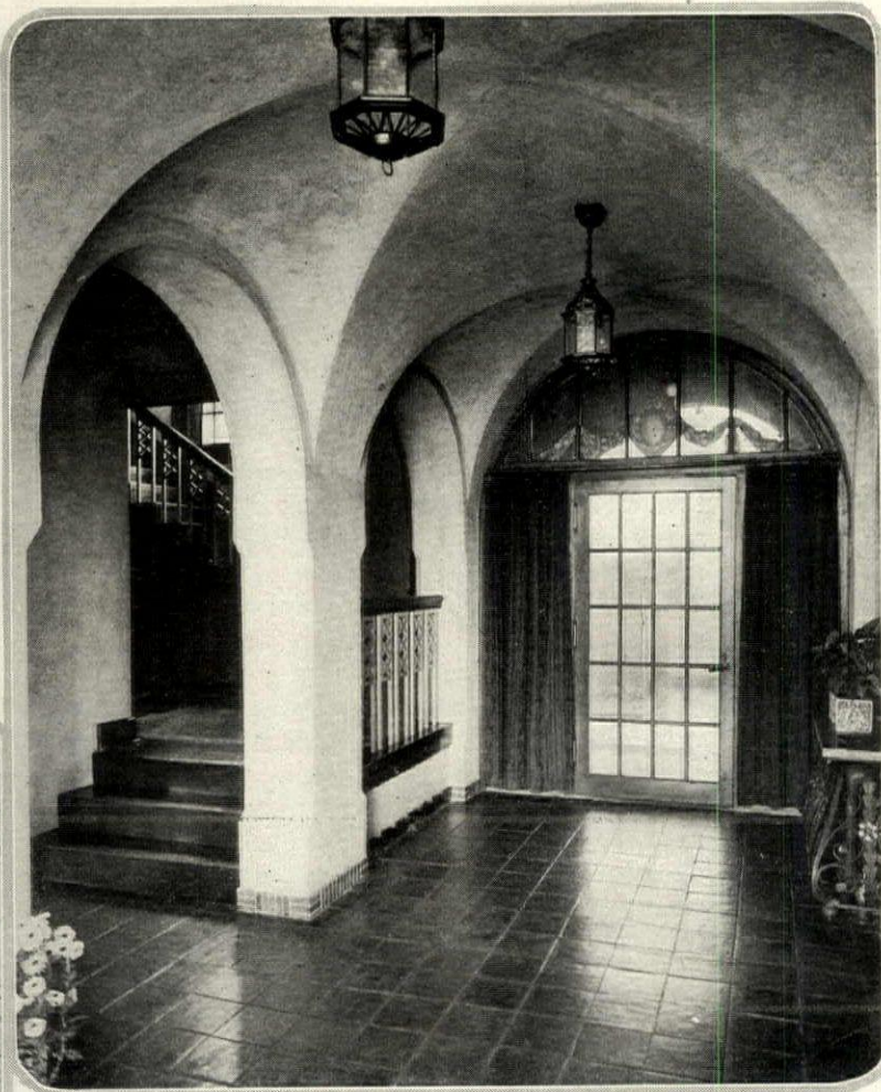
A hallway in which the architectural character both expresses and is expressed by the materials used, the plaster applied with a medium smooth trowelled finish. Howard Shaw is the architect
