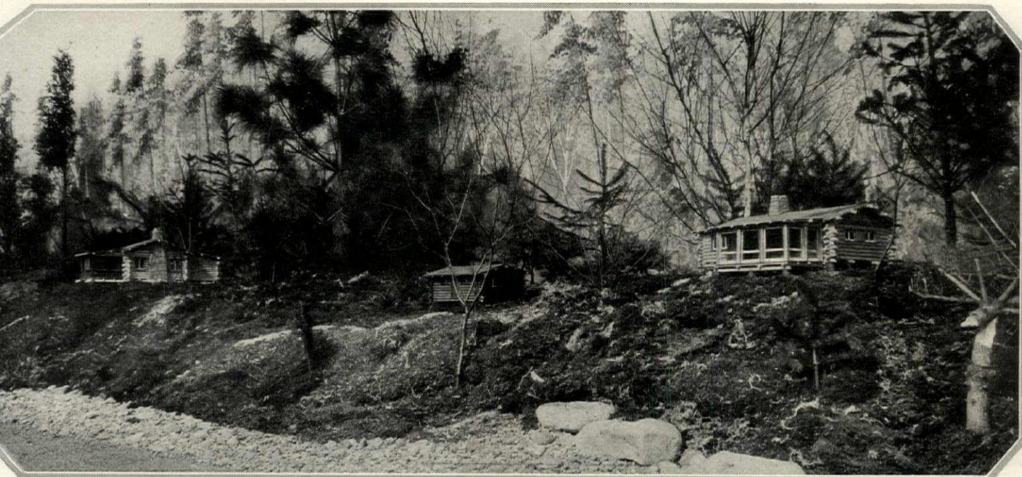
The site should be cleared of all trees which might fall athwart the cabin in a storm, but others should remain for shade and shelter. This photograph was taken from a model
