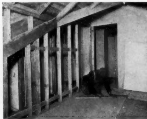
The various sorts of plaster or composition board are a reasonable and efficient substitute for plaster. They may be applied directly to the studding and, if battens are used over the joints, successful approximate paneling is realized. They are ready for use and need only painting, but the directions for cutting should be carefully followed
