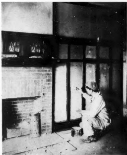
The various sorts of plaster or composition board are a reasonable and efficient substitute for plaster. They may be applied directly to the studding and, if battens are used over the joints, successful approximate paneling is realized. They are ready for use and need only painting, but the directions for cutting should be carefully followed
