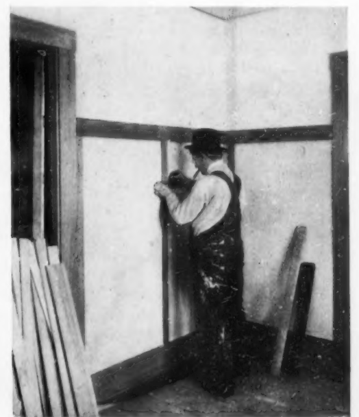
The various sorts of plaster or composition board are a reasonable and efficient substitute for plaster. They may be applied directly to the studding and, if battens are used over the joints, successful approximate paneling is realized. They are ready for use and need only painting, but the directions for cutting should be carefully followed
