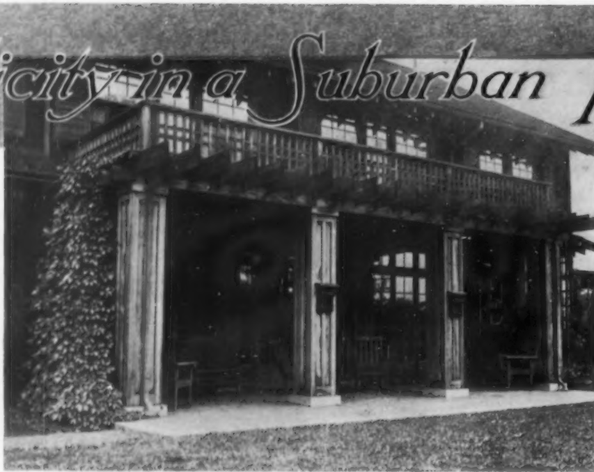
There is no fancy detail about the porches or the roof. The beams are left to show and are uncut and untrimmed
