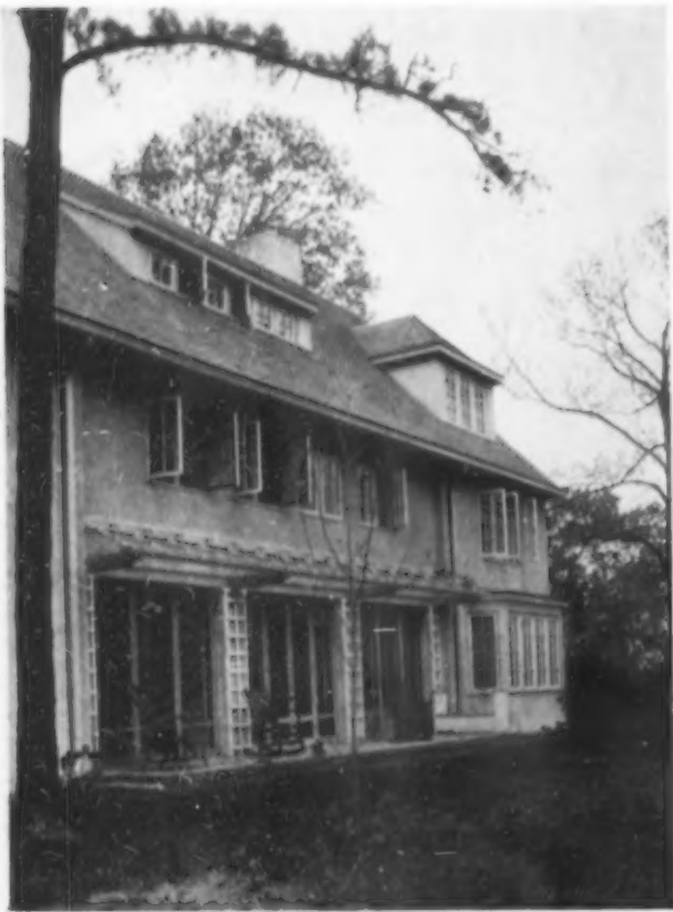
If the house is well sheltered, there is little necessity for a roofed porch; a lattice such as this is sufficient covering for the terrace
