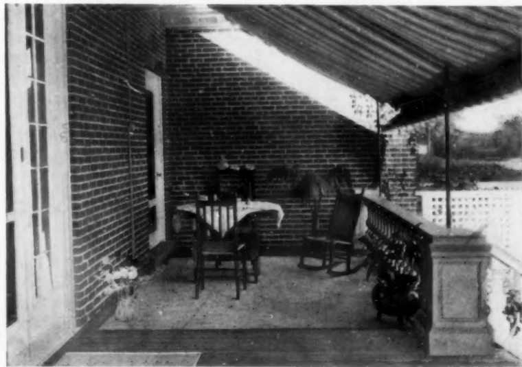
A terrace may be shaded or left open to the stars if its awning is arranged on an iron piping frame
