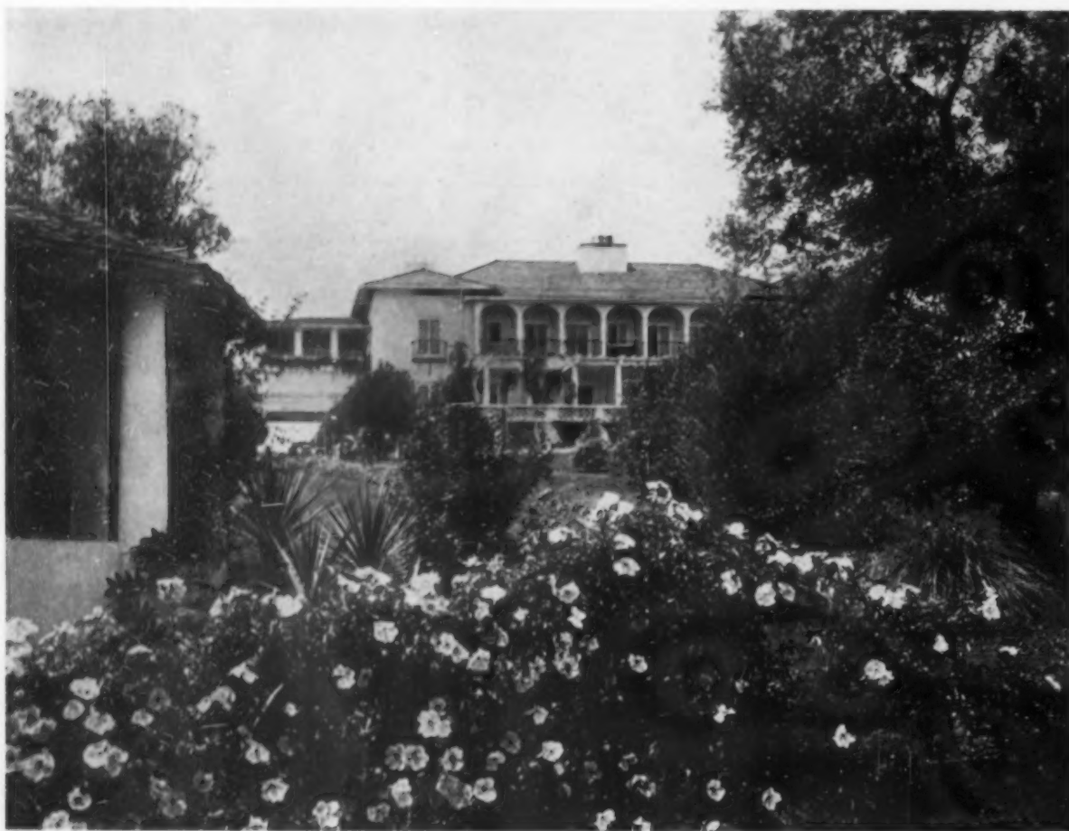
The house stands back from the street behind a hedge of roses and across a close-cropped lawn. Its walls are of white stucco over metal lath and the roofing is of shingles stained soft green
