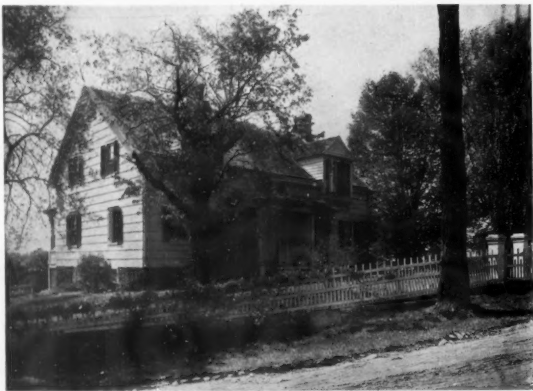
A natural effect has been gained here by placing the fence above a stone course set dry, and fitting the size of the fence to the increasing height of that course. Ramblers grown on the fence add a touch of color
