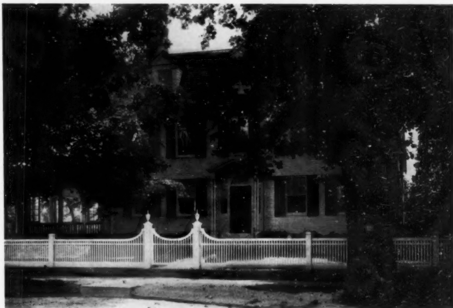
When the top of the gate is concave the terminal weight of the gates is lessened and the need for bracing eliminated. Aymar Embury, II, architect
