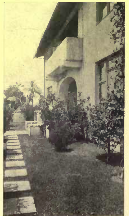
The impression of usefulness and strength visible in these houses is characterized by this sturdy balcony
