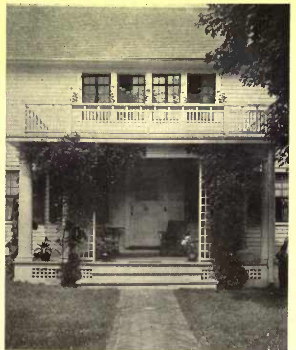
Hinged windows give access to the balcony from both of the front bedrooms
