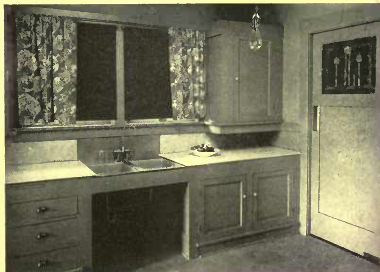
Concentrated efficiency—twin cobaltum sinks, sanitary vitrolite drainboard and work table, with flower bin and drawers below
