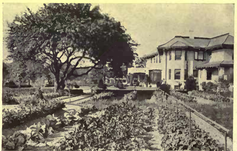
By running the pipe down the center of the garden both sides are reached, the mechanism being adjusted without labor
