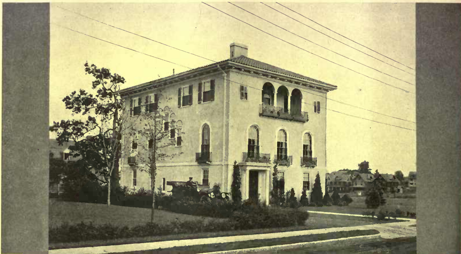
An Italian semi-suburban house, with all the floors above ground, saving space in the basement for garage, chauffeur's room, laundry and heating plant. In the front part of the basement are the entrance hall, library and reception room
