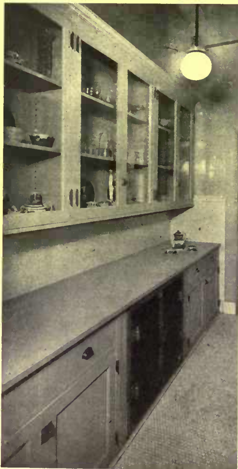
One of the new gas appliances is a plate warmer built into the cupboard in the butler's pantry
