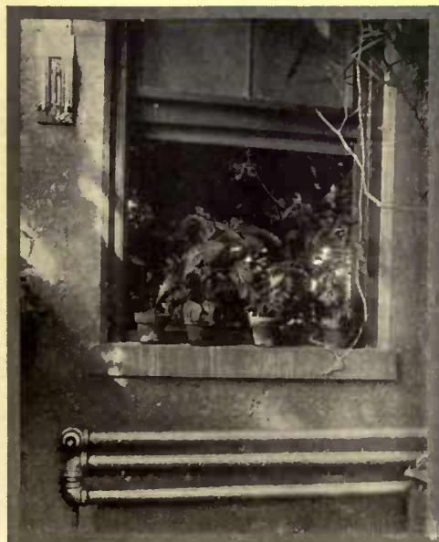
Extension from the steam radiator supplied sufficient heat and moisture to the air
