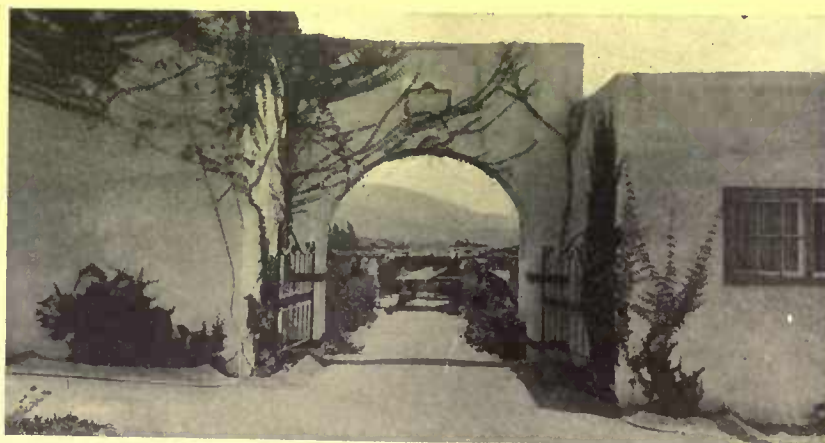
Concrete his medium; hollow tiles his walls. With these elements he constructs houses virtually time and fireproof
