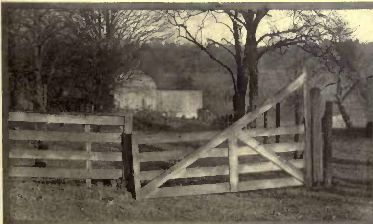
This is what generally happens—the post is none too heavy nor too well planted—and the gate sags
