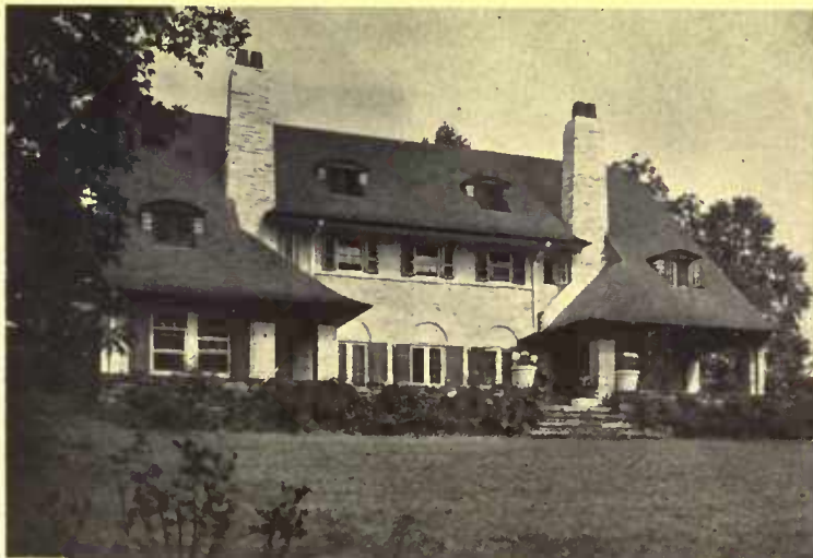
Dormers with arched hoods have been countersunk in the roof. Square, white chimneys with red pots lend color
