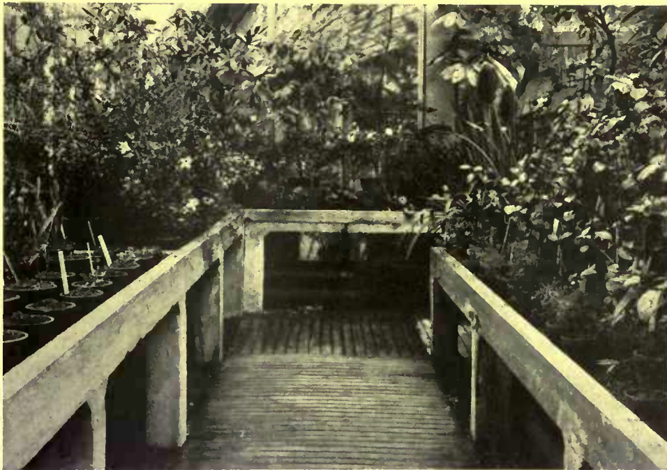
In the greenhouse the possibilities of concrete are almost limitless. No material is better for shelves, supports and flooring
