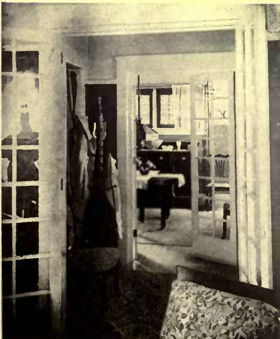
A view across the hallway to the dining-room, showing the use of double full light doors
