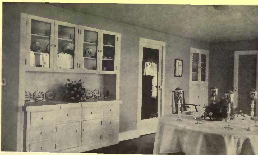
Here, in his almost elimination of wood, the door frames and windows are sunk flush with the wall
