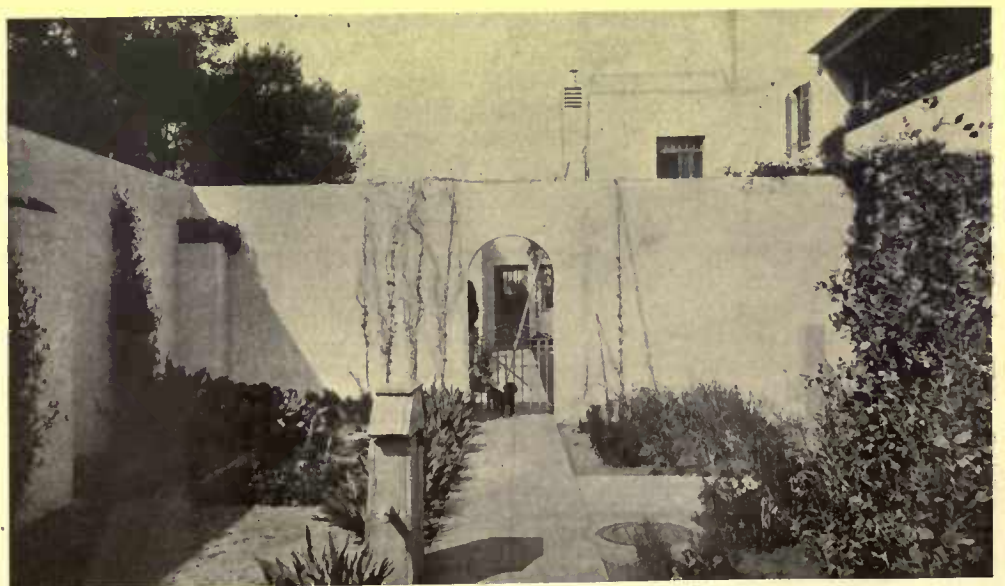
High walls pierced by arched gates, providing privacy to rear gardens and balconies, are a pronounced detail
