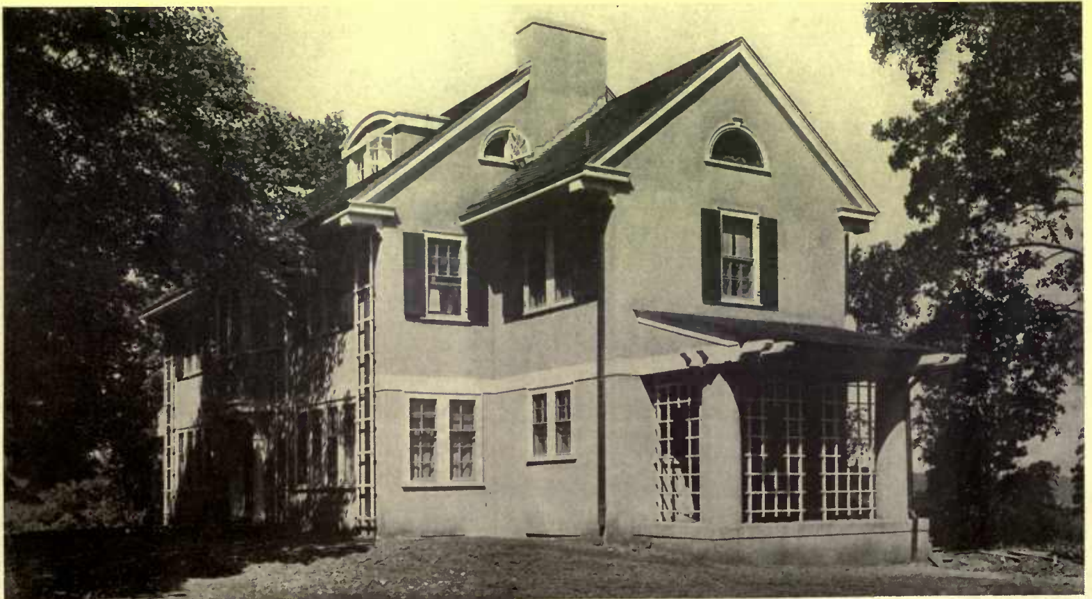
The service porch has a cement floor and is screened with a lattice both practical and decorative. It affords easy access to the built-in refrigerator and an unbroken passage for the ventilation of the kitchen itself
