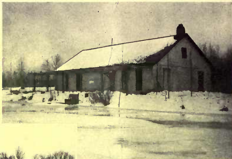
The heavy walls had to be pierced with long windows and doors
