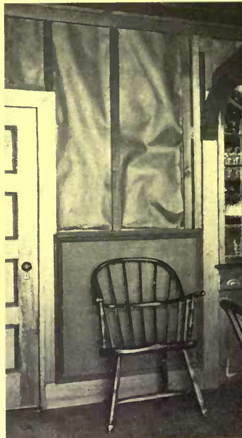
In instances such as this panel board is the best solution against the dampness
