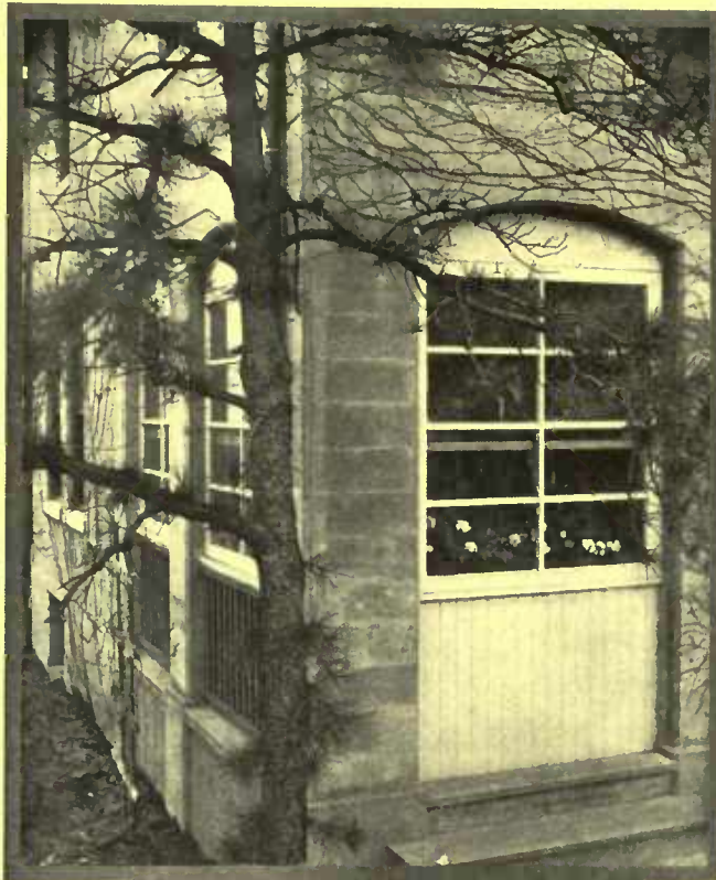
Showing the simple manner in which the porch was enclosed and how readily it can be thrown open for summer use
