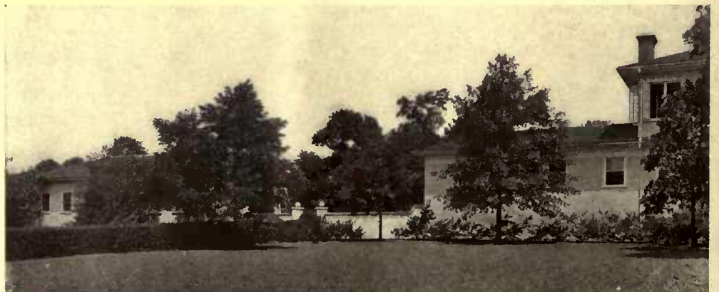
Gray stucco walls separate the service quarters from the gardens and carry the lines of the house itself to those of the garage and lodge
