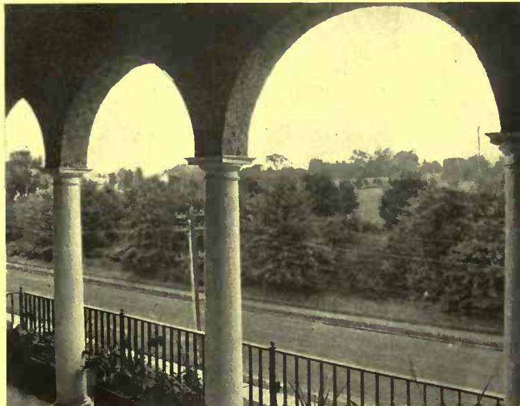
Ample piazza room has been obtained by recessing to form loggias, providing shade and privacy, and in winter permitting an enclosure
