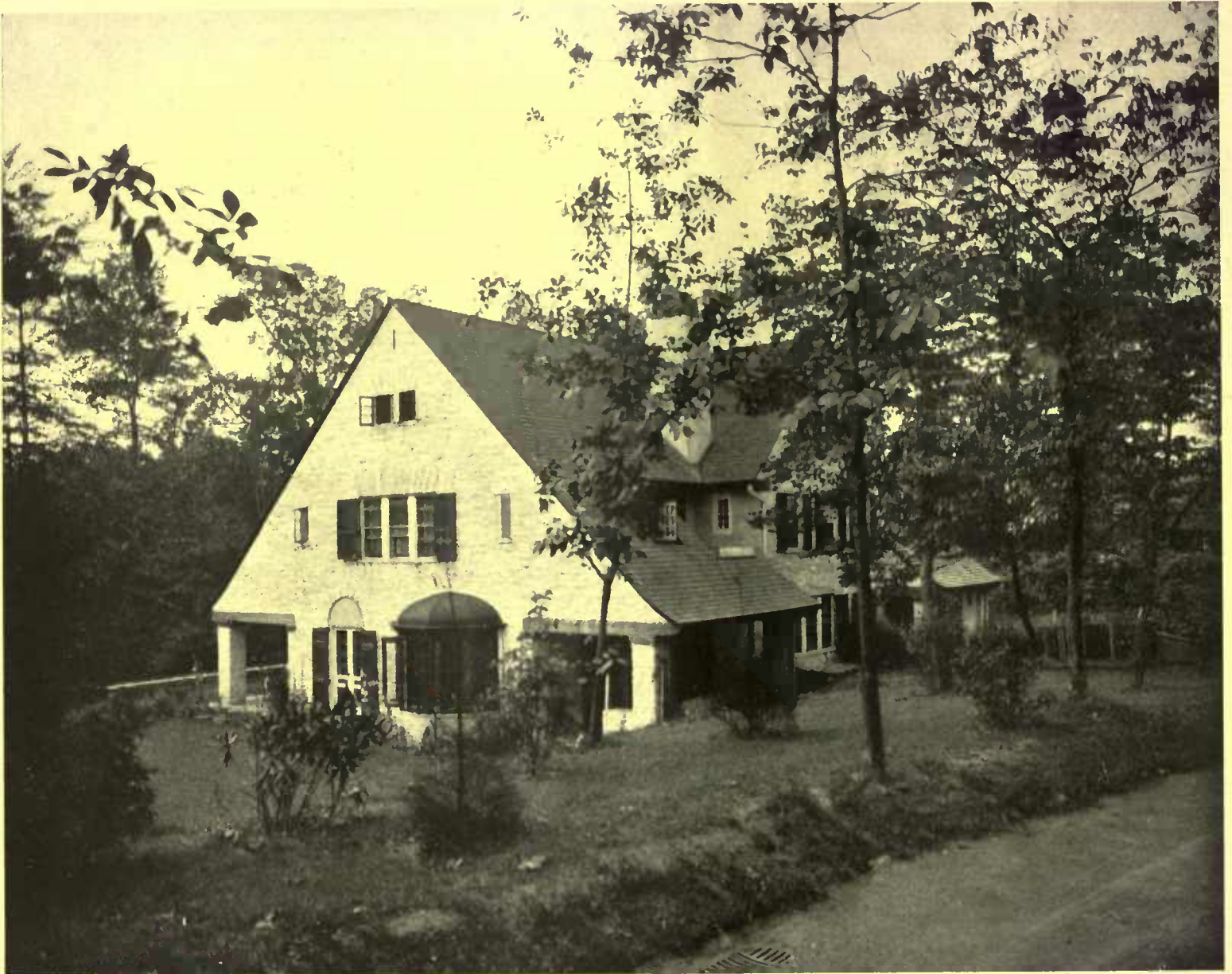
Several problems were involved in the site, which is on a steep western hillside, with a roadway at the top. These were met by backing the house to the entrance with the front to the west, and building low and snug along the ridge with native materials
