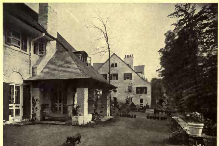
The house sits down well on the ground, as it ought. At the eaves the roof has a little flaring kick-up
