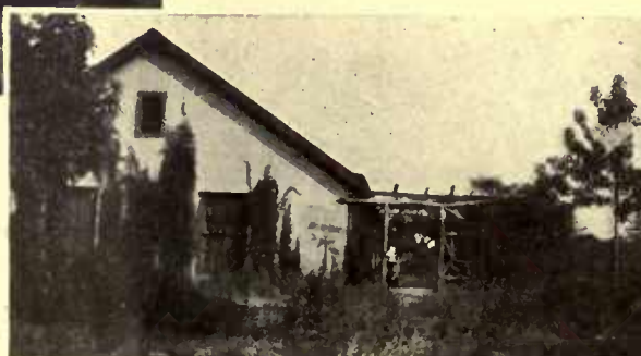
After the grading, vines were run up the walls. Voila!
