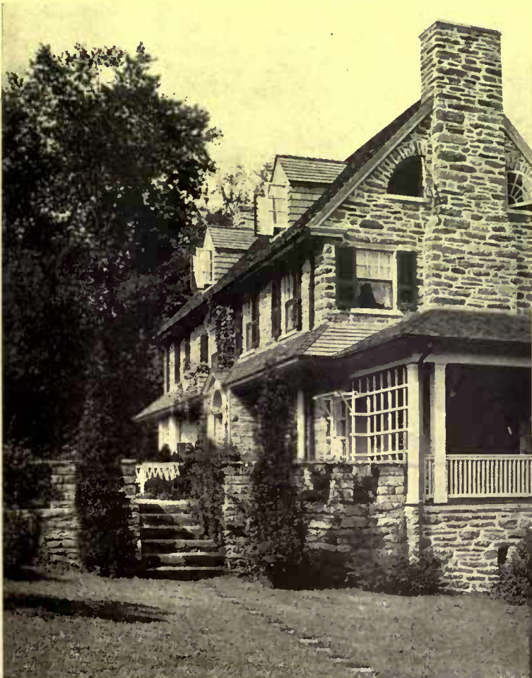
An especially good color has been obtained by the rubble walls of quarry stone
