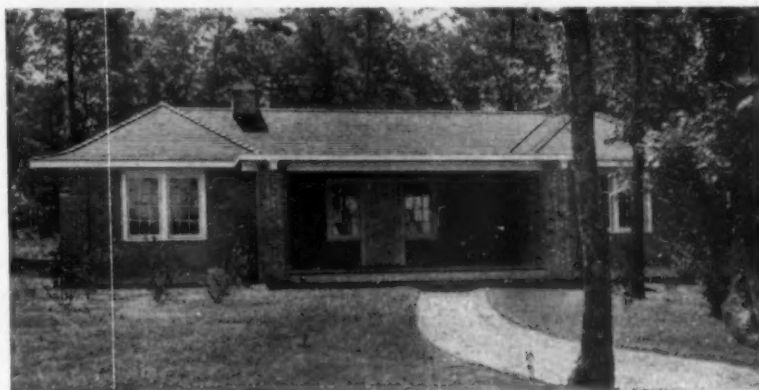
An interesting combination of brick piers and plaster on wood frame, at Belle Terre, L. I. Aymar Embury, architect
