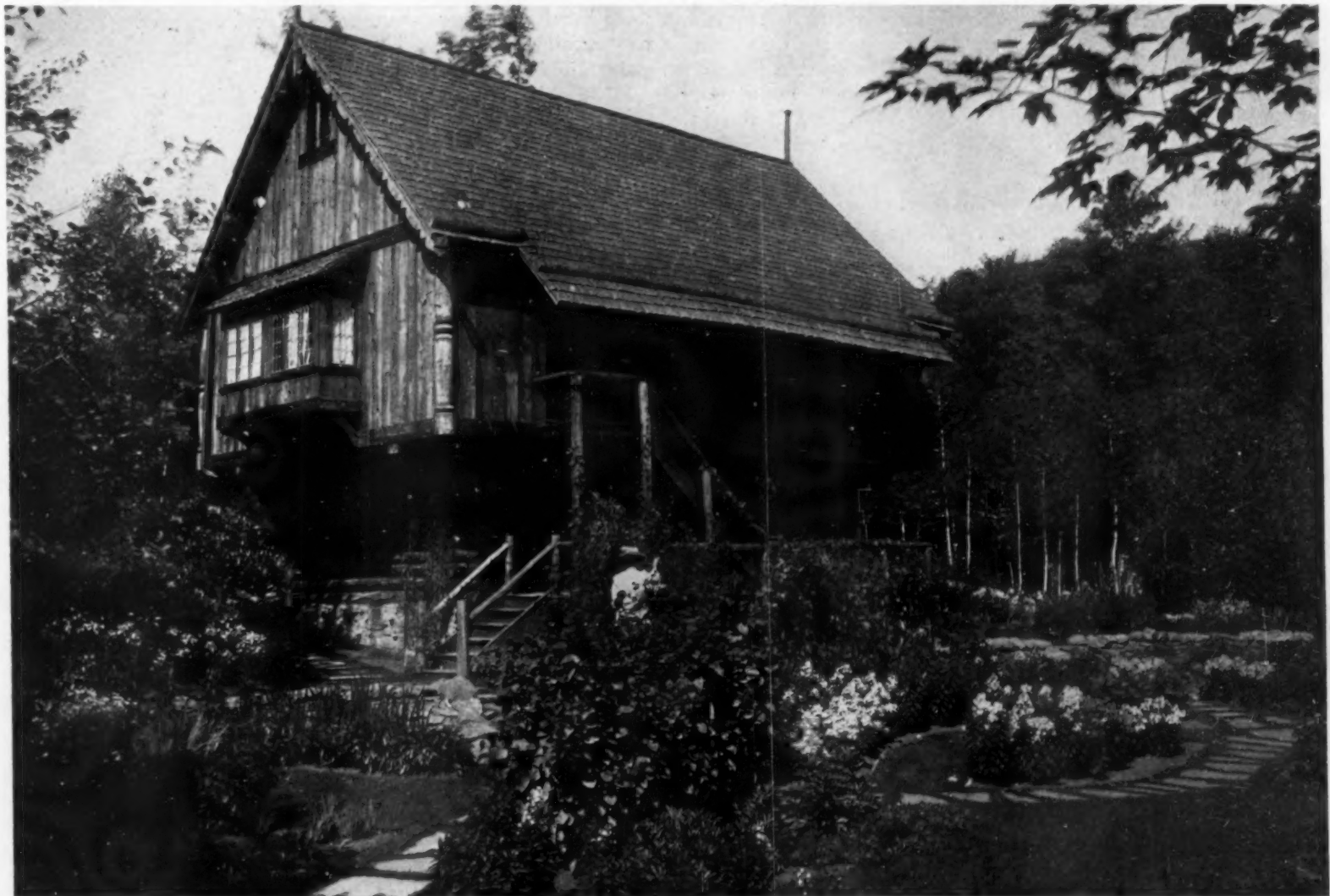
Spruce logs were used for the first-story walls, with uncolored oiled woodwork above, and a roof of hemlock slabs. George A. Reid, architect
