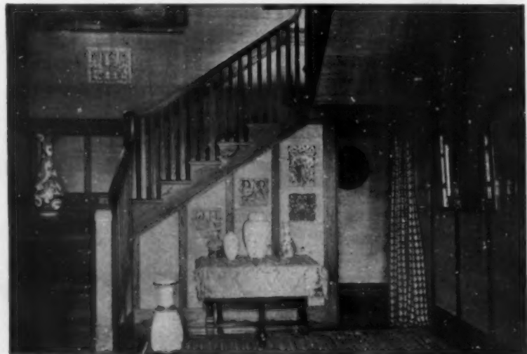
The woodwork in the first-story hall is chestnut, stained brown, the wall covering between the panels being gold grass cloth
