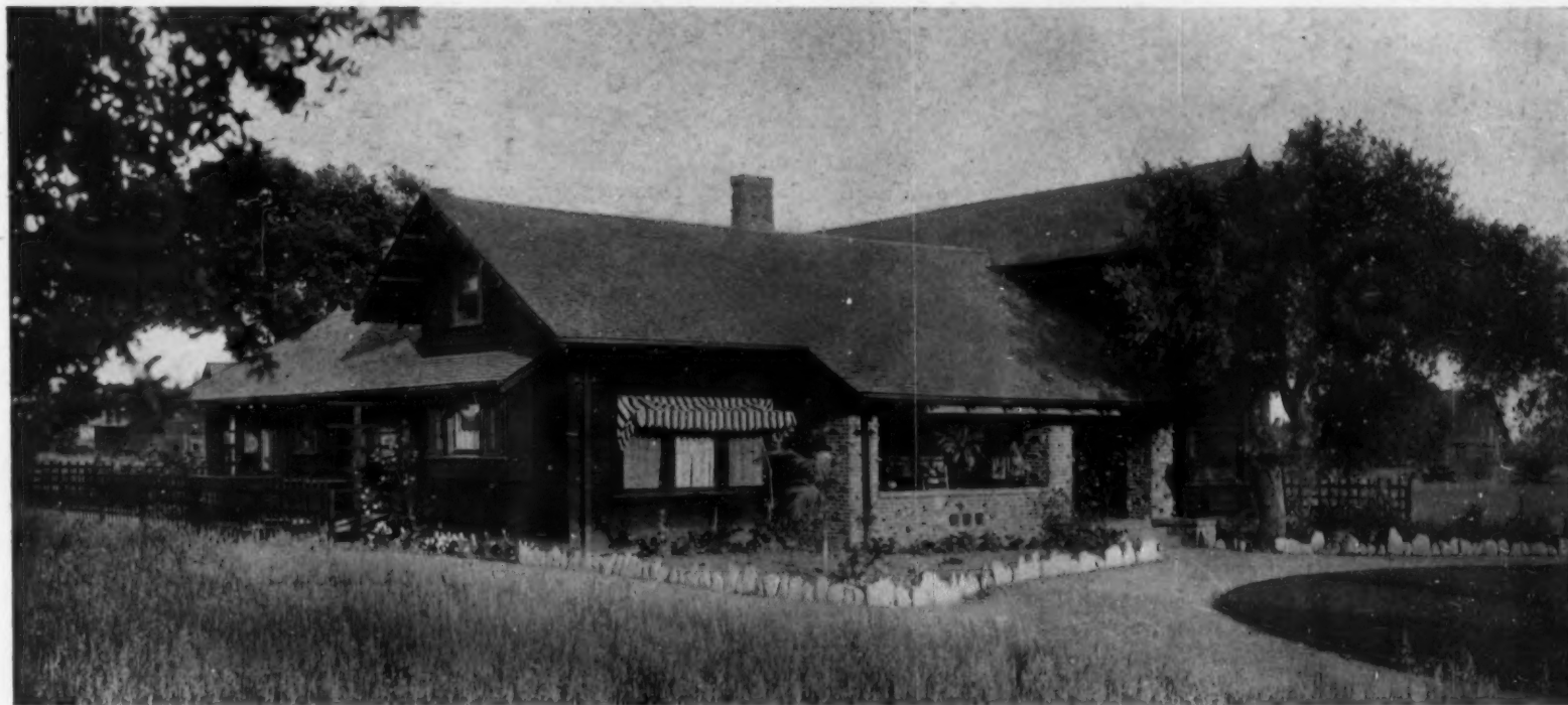
A bungalow at South Pasadena, Cal., built of redwood shingles and brick that is interspersed with clinkers. The floor plan appears below. Lester S. Moore, architect
