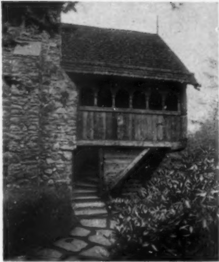
An outside stairway leading to the studio proper shows characteristic Norwegian detail
