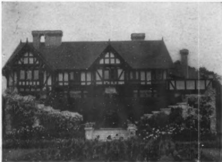
Kelsey Heated, at Germantown, Pa. Mr. Oswald C. Hering, Architect. IN NO OTHER FIELD HAS THE KELSEY FRESH AIR SYSTEM SCORED GREATER SUCCESS THAN IN THE HEATING OF LARGE FINE COUNTRY HOMES.
