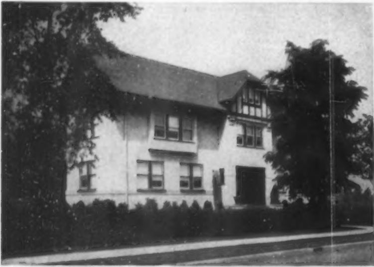
"Garden Corner" is built of stucco on a wood frame. The exterior woodwork is of cypress stained brown; the hinges are silver gray; the sash, sage green
