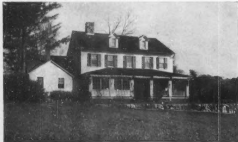
The rear of the same house. The long porch, glazed-in in winter, commands the view over the meadows
