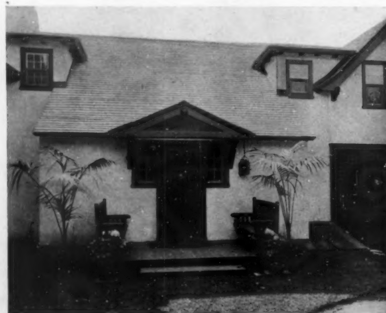
The entrance door, with its projecting hood and flanking seats, opens into a vestibule coat-room
