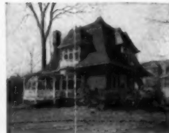
A No. C-241 IDEAL Boiler and 555 ft. of 3/8-in. AMERICAN Radiators, costing the owner $260, were used to Hot-Water heat this cottage.
