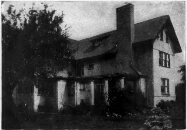
The only porch on the house is in the corner formed by the ell and sheltered from the sun by a vine-covered pergola motive, giving a view over the garden
