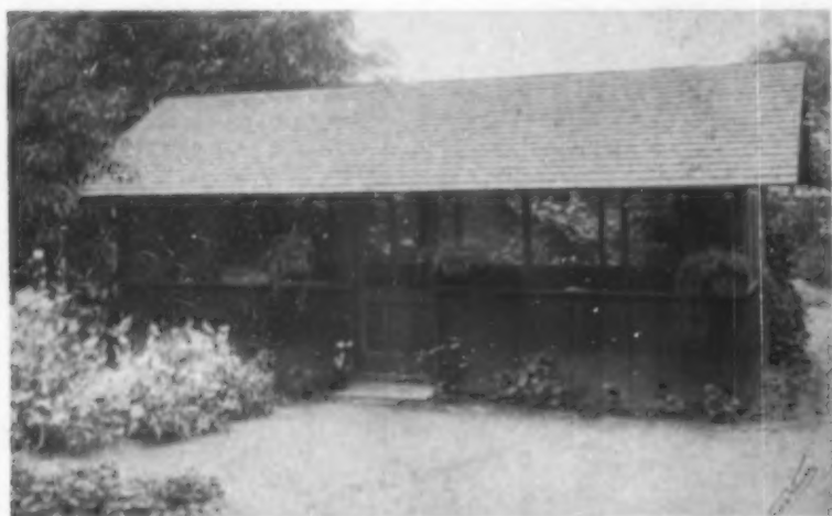
If you cannot get away for the Summer you can build a sleeping-room in the garden
