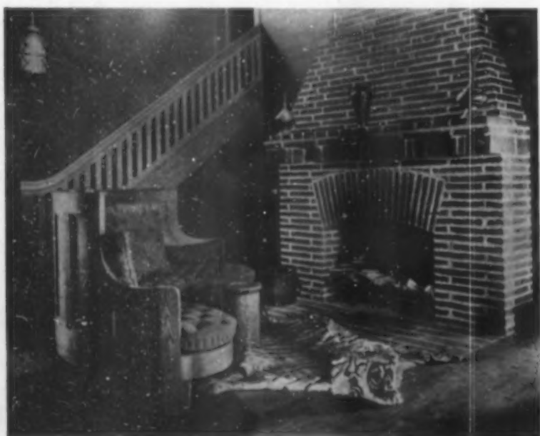
A great rough-textured brick fireplace, laid with broad white joints stands at one end of the living-room
