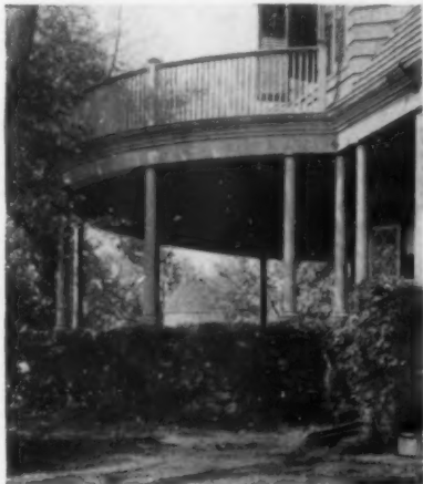
If one can swing out a generous octagonal or circular corner, comfort is gained with less darkening of the first-story rooms
