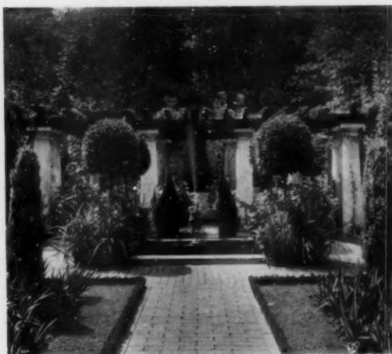
Of all pergola types that modern ingenuity has developed, the combination of white plaster columns with dark creosoted beams is probably the most effective
