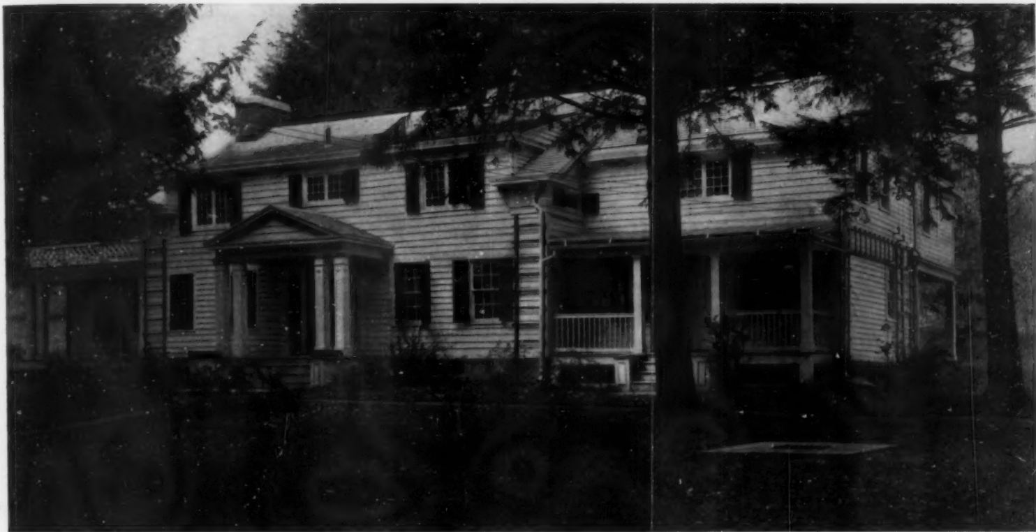
The front of the house was made lighter inside by removing the long front veranda, shown in the picture below, using the old columns and moldings of pure Greek contour in a simple entrance porch at the front door
