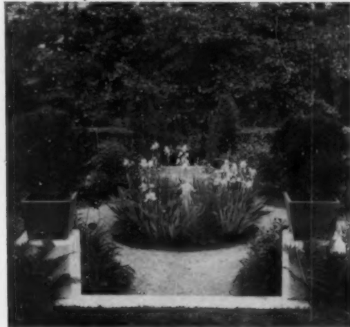
Steps and flanking pedestals for formal plants may easily be made from cement
