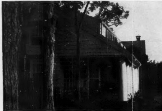
Mr. Chauncey Olcott's home at Saratoga Springs shows the modified Dutch Colonial type, where the long sweep of the roof comes down to cover the porch. Keen & Mead, architects
