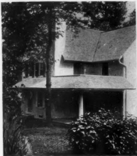
An interesting corner porch, with an upper balcony and a Germantown hood. George Spencer Morris, architect
