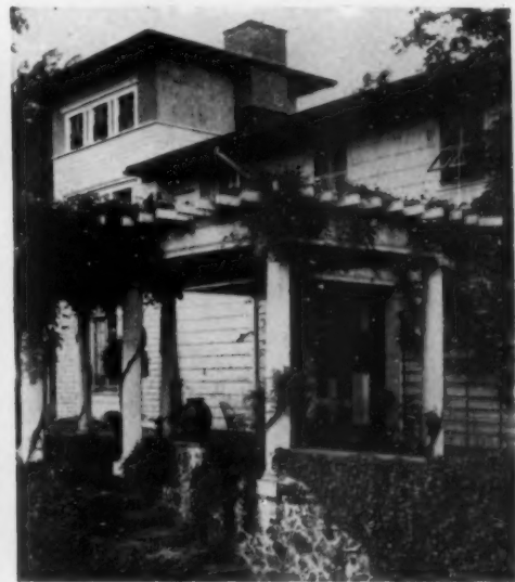
It is becoming increasingly common to have either an uncovered terrace or one that is shaded by a pergola
