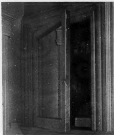
A medicine closet in a partition that is roomy enough to hold large bottles
