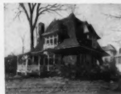
A No. C-241 IDEAL Boiler and 555 ft. of 38-in. AMERICAN Radiators, costing the owner $250, were used to Hot-Water heat this cottage.
