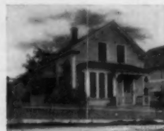
A No. 3-25 IDEAL Boiler and 400 ft. of 3/8-in. AMERICAN Radiators, costing the owner $195, were used to Hot-Water heat this cottage.
