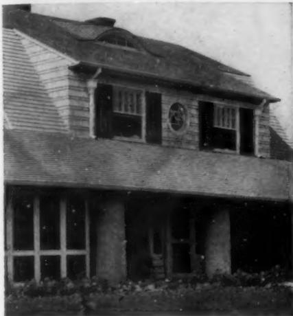
The circular window ventilates a closet, the "eyebrow" window above lights the attic
