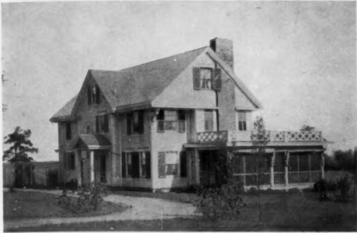
Clapboards in most localities make the cheapest wall in a first cost, but the repainting brings up the total
