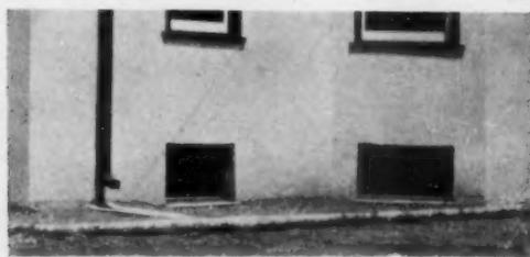
Lead the water from rain conductors away from the foundations
