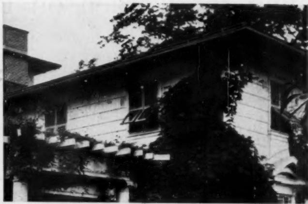
This scheme of double-hinged blinds cuts off the sun without keeping out the air
