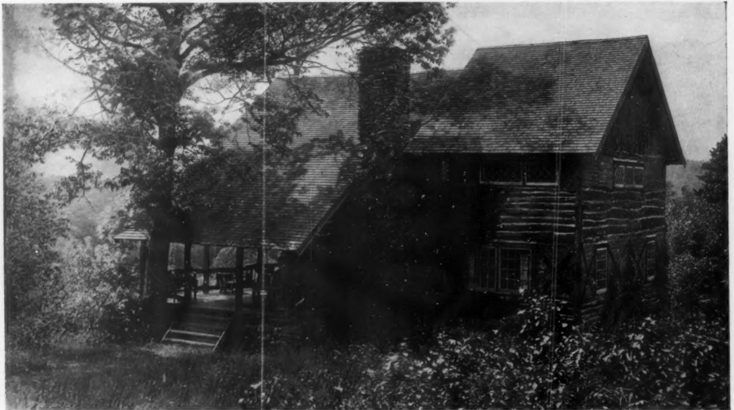
The outside cuts from chestnut logs were nailed to an ordinary stud frame, the chinks being filled with cement on wire mesh
