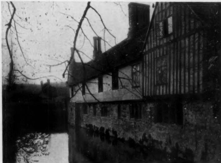
Much of the charm of old half-timber houses results from the use of various materials in combination and in the looseness of construction—notice for instance the uneven spacing of the gable-end timbers
