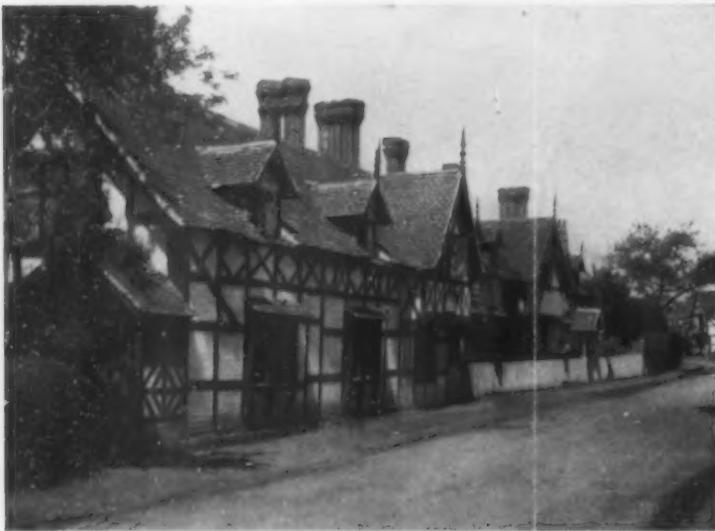
Half-timber walls are not always of timber and plaster; bricks have been used here for the filling or "nogging"
