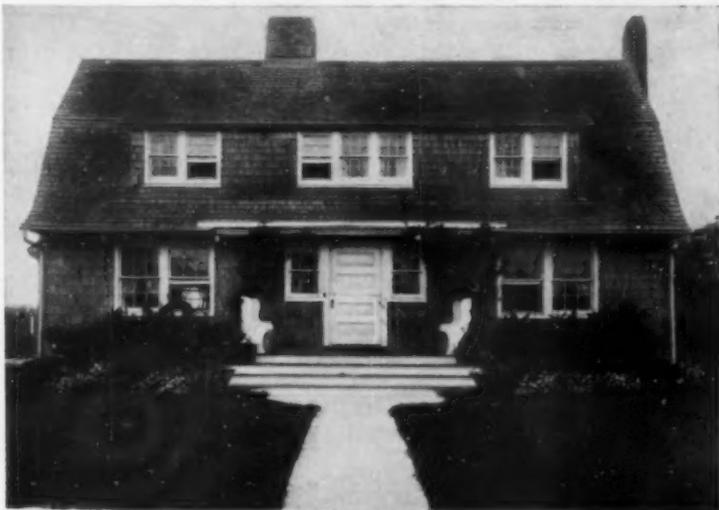
Shingles for walls have a reasonably long life, particularly if dipped in a creosote shingle stain before being put on
