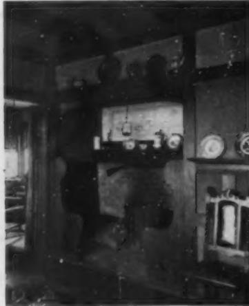
The seats here are rather too close to the fire for comfort. Make the inglenook seats of box form, with hinged lids, so as to have a convenient space for firewood
