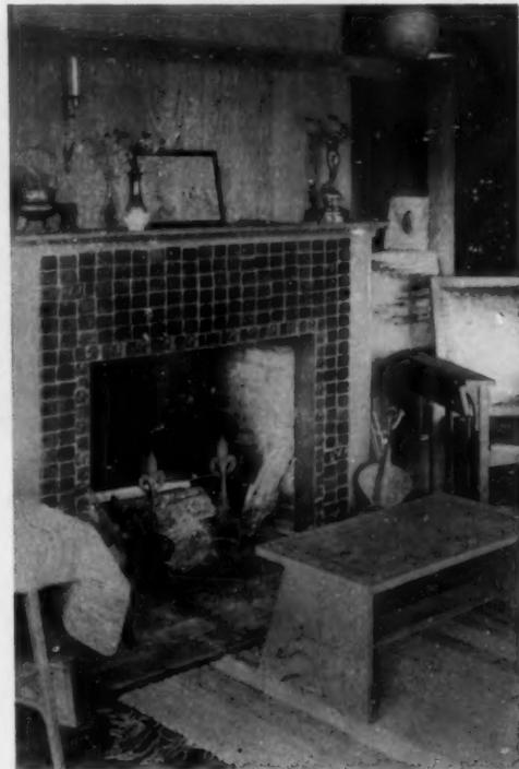
Small, dull hand-made tiles make a charming facing for the fireplace and may be set in cement over unattractive brickwork
