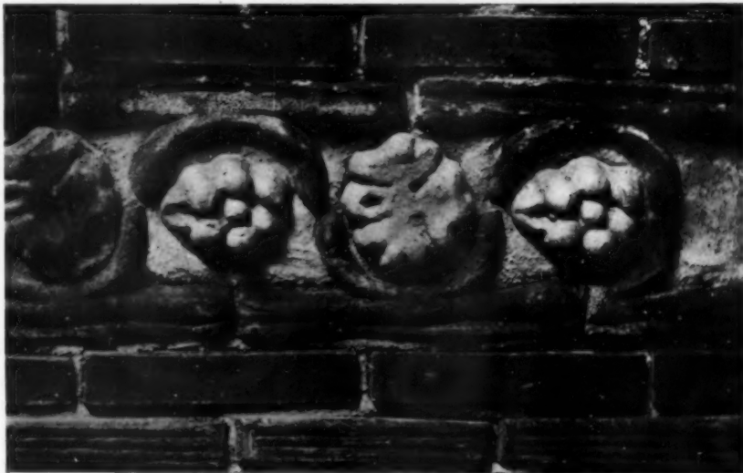
Fig. 5. A border consisting of relief tiles in silhouette banded with flat rectangular tiles, the whole representing a grape vine with fruit and leaves in three repeating units of pattern. Tiles are set in light cement plaster. The cement background is freely used as part of the design. The central tiles are pushed into the wet concrete. Colors: red, green, blue, black, gray and buff
