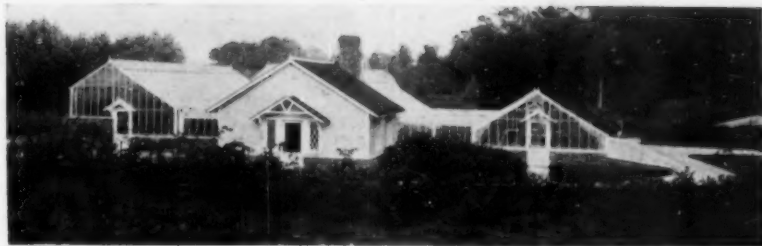
From the work room side it is specially attractive
