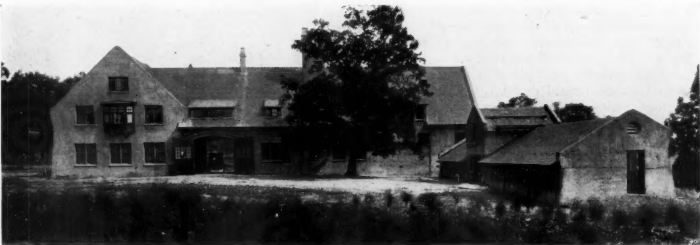
PRIVATE STABLE AND POULTRY HOUSE ON THE PABST ESTATE
