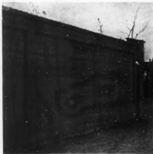
Fig. 8. Another style of concrete fence or wall with tile coping
