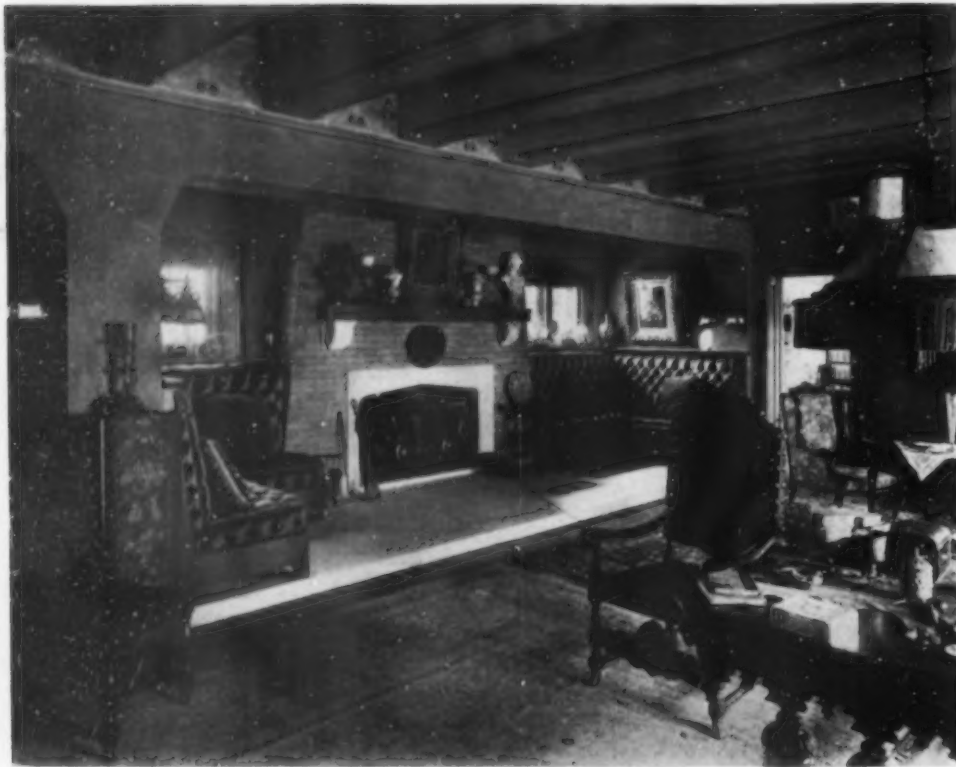
THE FIREPLACE IN THE LIVING-ROOM Note the reinforced concrete beams
