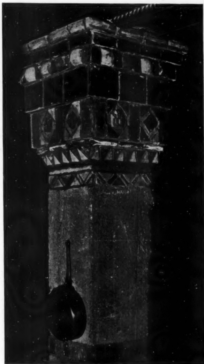
Fig. 2. Column of Byzantine pattern in original unplastered concrete, supporting heavy ceilings. Capital ornamented with colored tiles, glazed and unglazed, flat and in relief. Colors: yellow, green, blue, gray, red, white and buff
