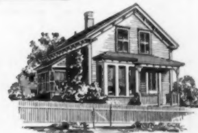
A No. 015 IDEAL Boiler and 175 ft. of 38-in. AMERICAN Radiators, costing the owner $116, were used to Steam-Heat this cottage, at which price the goods can be bought of any reputable, competent Fitter. This did not include cost of labor, pipe, valves, freight, etc., which installation is extra and varies according to climatic and other conditions.
