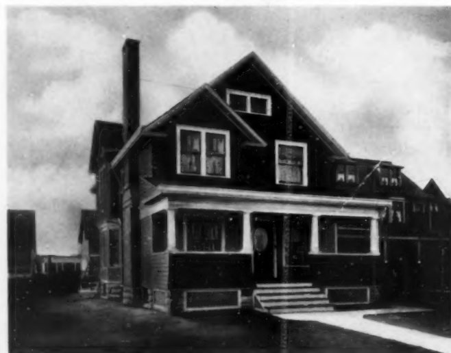
A TYPICAL OHIO HOME Warmed by a Water Plant costing $300
