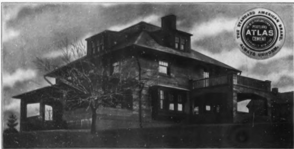
A Concrete Residence at Briarcliff Manor, N. Y. A. G. Richardson, Architect
