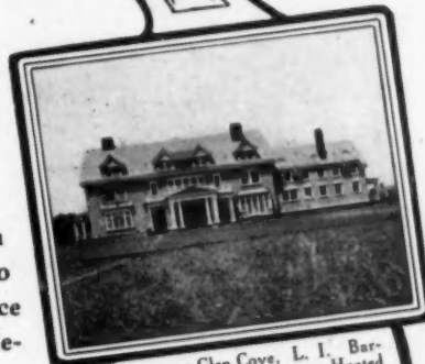
Residence at Glen Cove, L. I. Barney & Chapman, Architects. Heated by the Kelsey Warm Air Generator.
