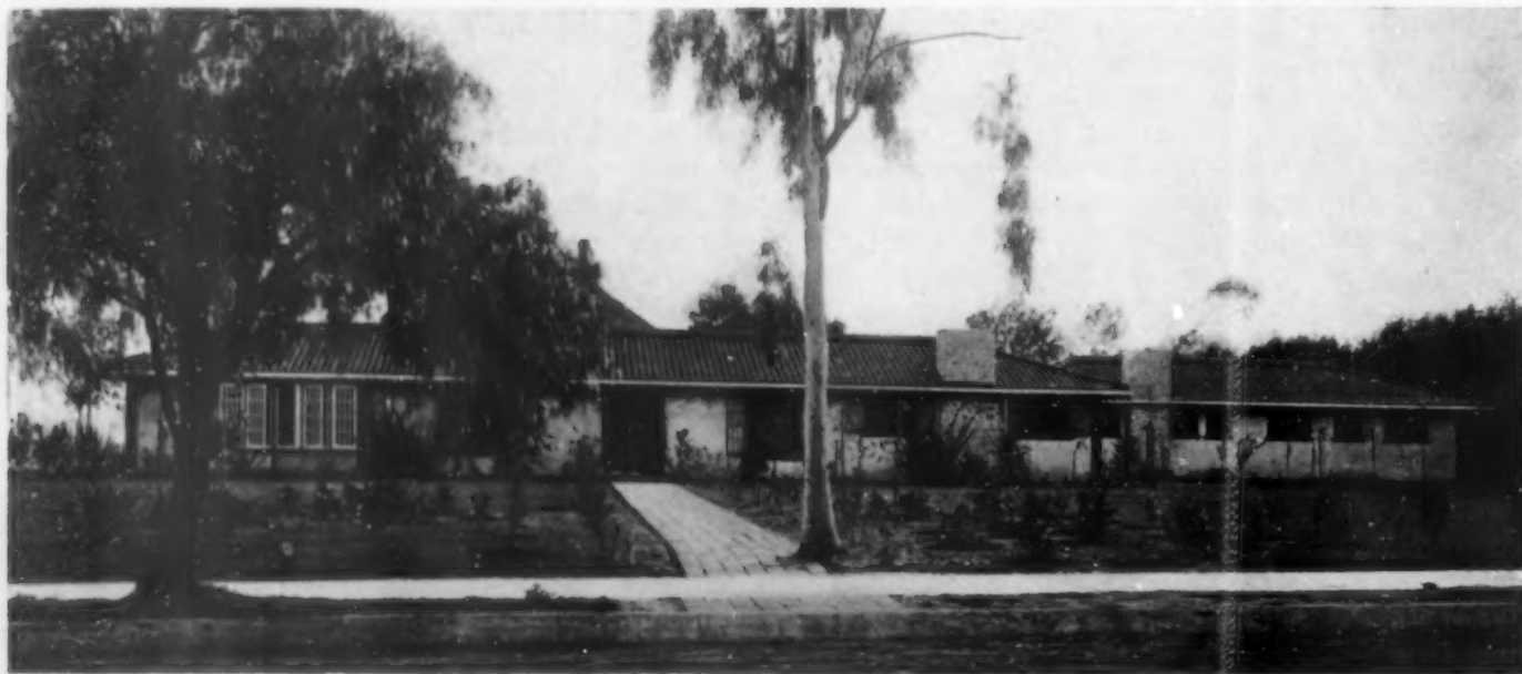
THE HOUSE OF MR. A. J. EDDY, PASADENA, CALIFORNIA, SHOWING MEXICAN INSPIRATION
