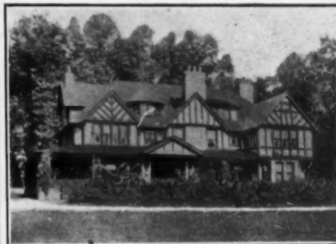
Kelsey Heated Residence, Ardmore, Pa.
