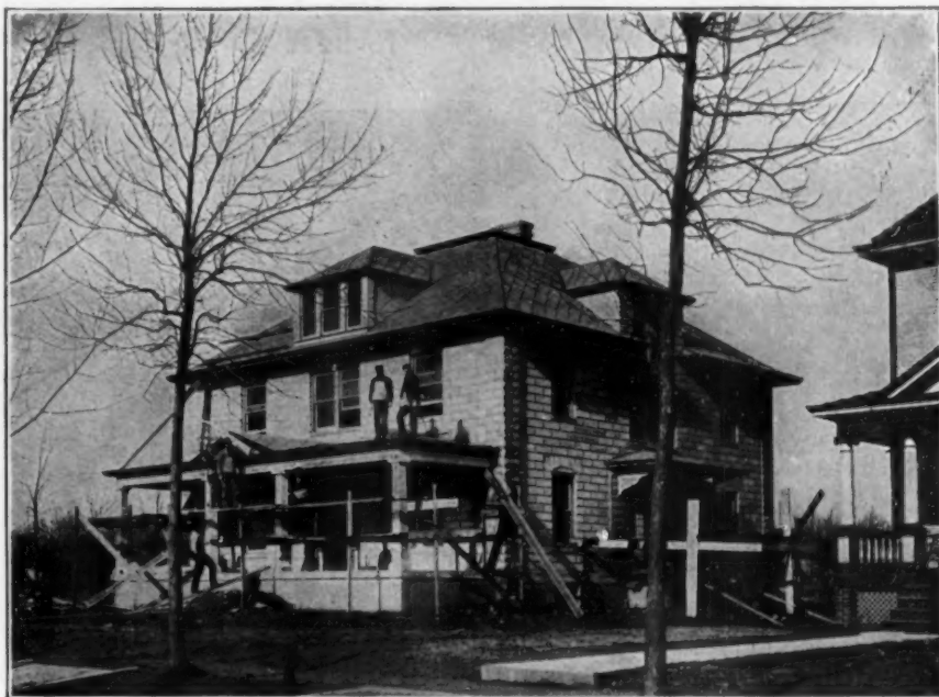
Illustrating a Concrete Block House of Dr. H. C. Howard, Champaign, Illinois, Prof. F. M. White, Architect, roofed with Asbestos "Century" Shingles, laid French Method.
