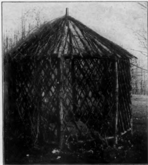
A LATTICE-WORK HOUSE
