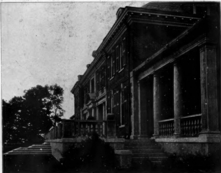
THE UPPER TERRACE FROM THE EAST
