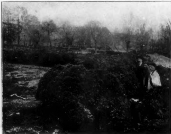
THE TRENCH BESIDE THE HEDGE
