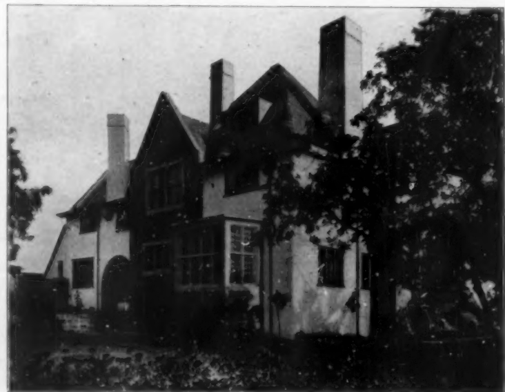
A HOUSE AT KENILWORTH The North Front
