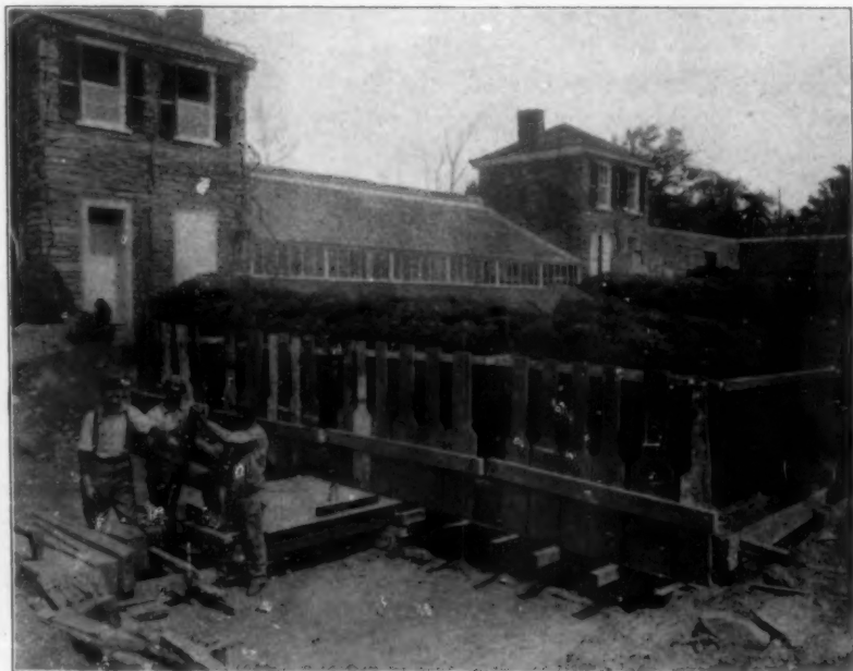
FORCING IRON PLATES UNDER THE ROOTS
