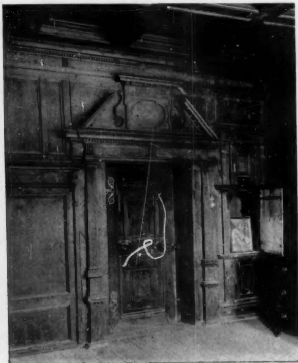
INTERIOR AT ST. MICHAEL
