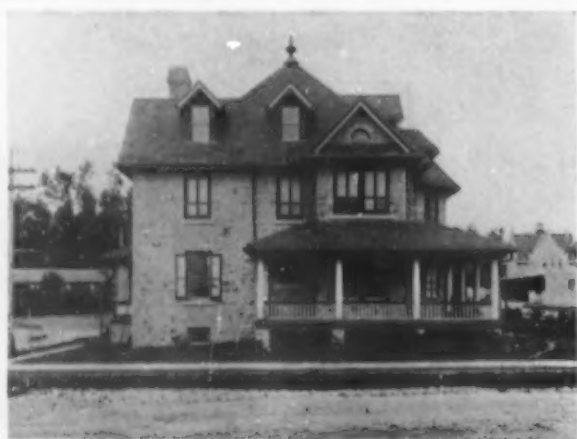
RESIDENCE FOR RICHARD V. MATTISON, AMBLER, PA. MOTTLED WAVE TILE WITH RHINOCEROS TILE AT EAVE LINE MEADE ROOFING & CORNICE CO., Contractors
