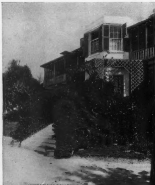
ENTRANCE TO AN OFFICER'S RESIDENCE
