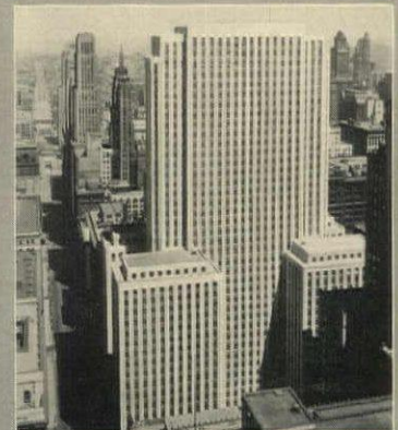
Marshall Field Building, Chicago—Graham, Anderson, White and Probst, Architects
