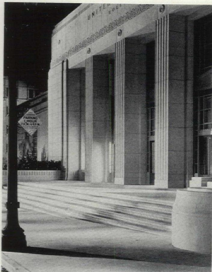
HOLLYWOOD, CAL., POST OFFICE. ALL CONCRETE BLDG.
