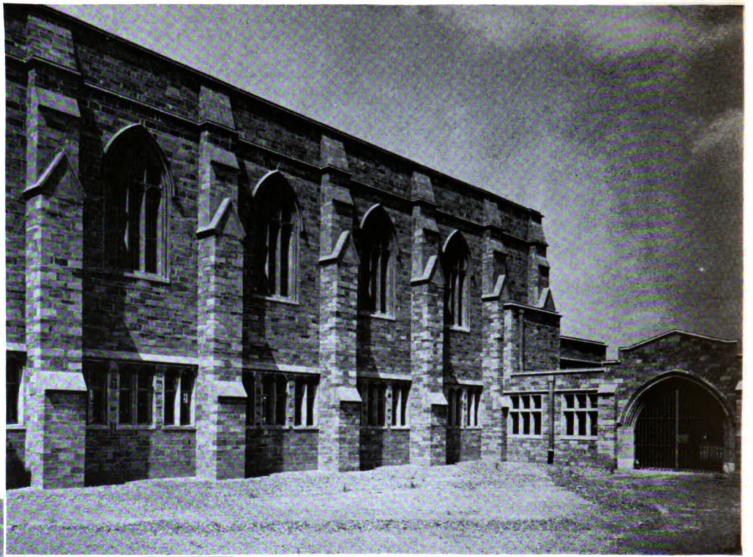
Berks County Prison, Reading, Pennsylvania. Coursed concrete ashlar, built with colored and textured units, is the basis for the architectural interest in the walls of this building. Alfred Hopkins and Associates, Architects.
