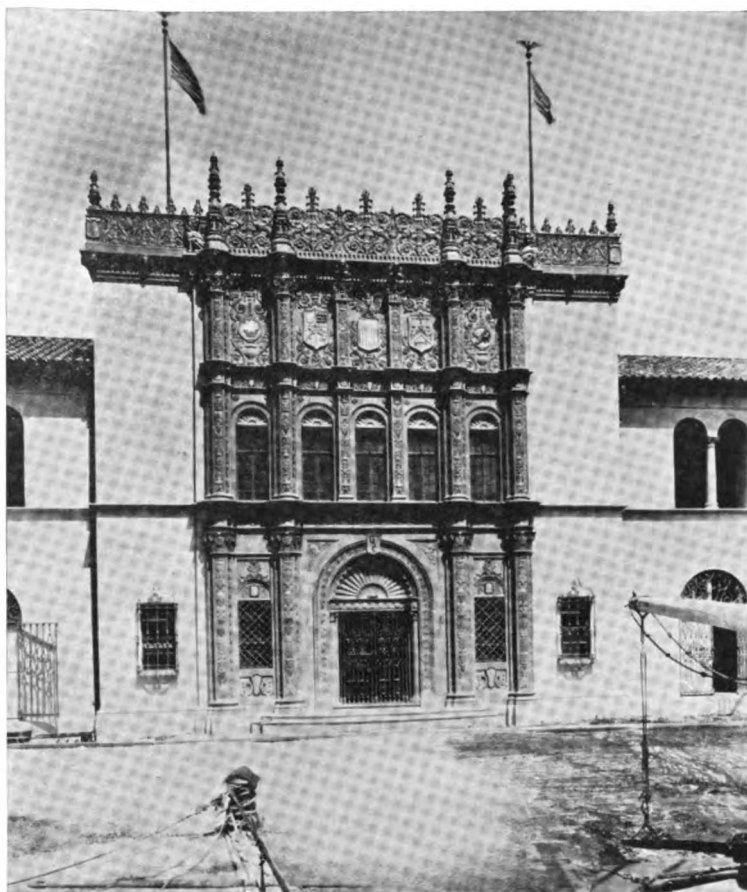
UNITED STATES CUSTOM HOUSE, SAN JUAN, PUERTO RICO Albert B. Nichols, Architect J. C. Besosa, Builder
