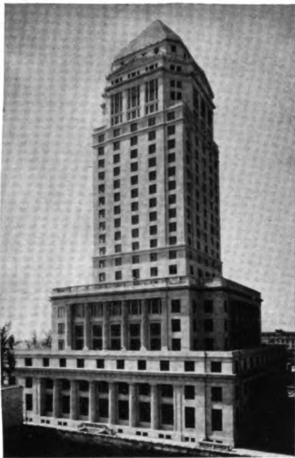
Miami City Hall and Dade County Courthouse, Miami, Fla. Entirely faced with Atlantic Terra Cotta.
