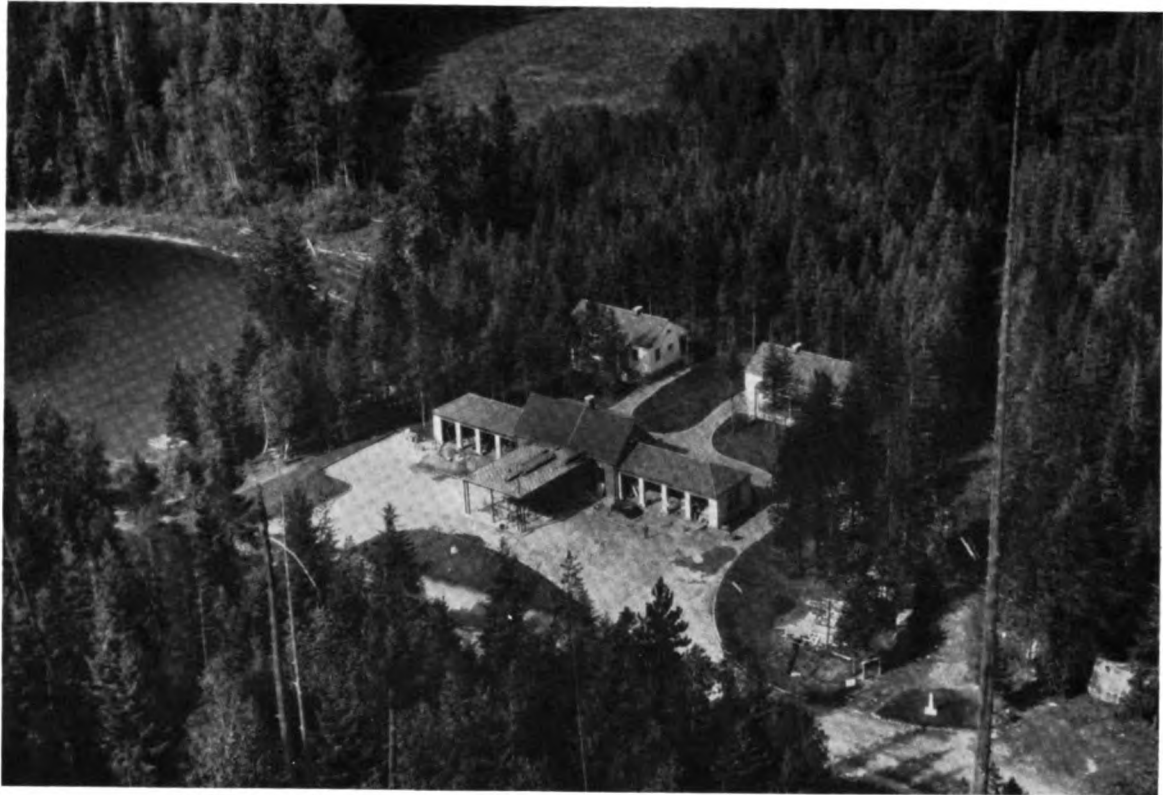
METALINE FALLS, WASHINGTON INSPECTION STATION
