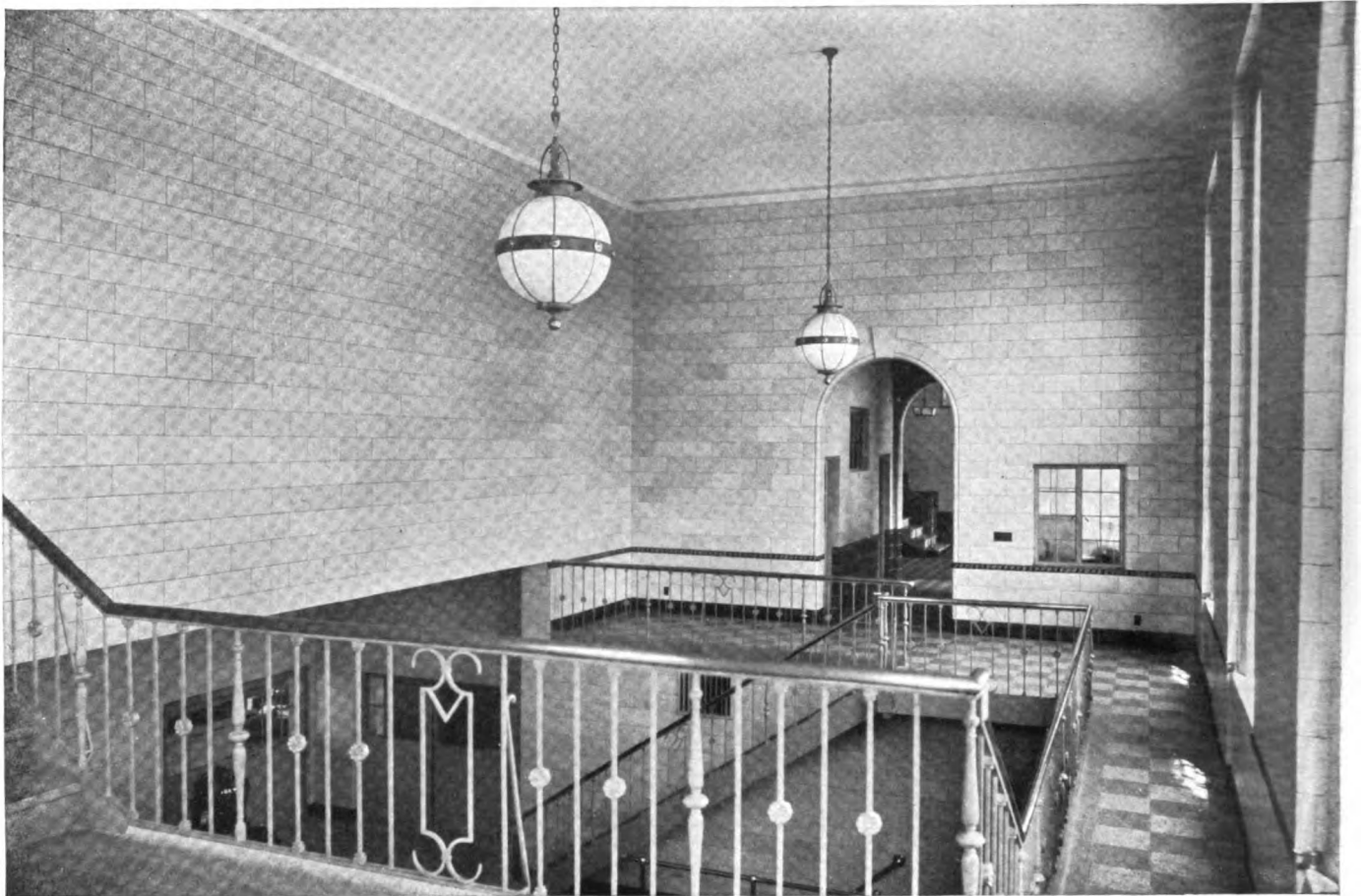
Disposal Plant—Dearborn, Michigan; Architect—Hubbell, Hartgering & Roth; Builder—W. H. Mueller Co. The lobby, passage ways, offices, motor room and laboratory are faced with Federal Seaboard Wall Ashlar.
