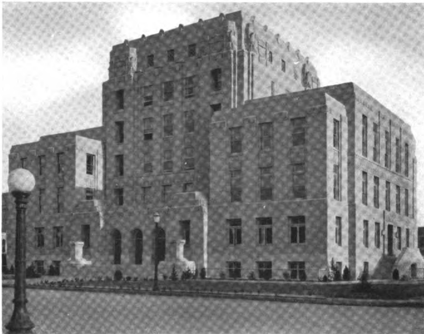
Eastland County Court House Eastland, Texas
