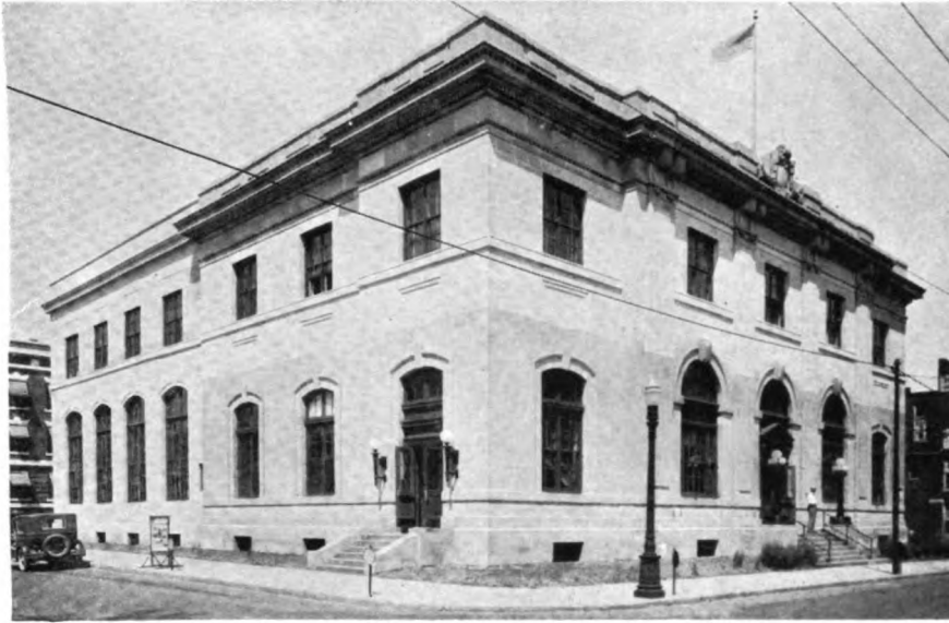
U. S. Post Office Anderson, Indiana Exterior of Limestone from Victor Oolitic Quarry, cut by the Carl Furst Company.
