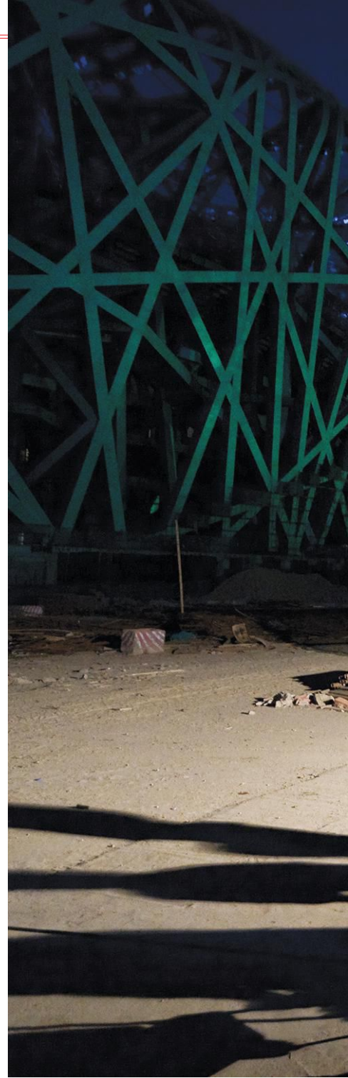
National Stadium, by Herzog &amp; de Meuron. Beijing, 2007.
