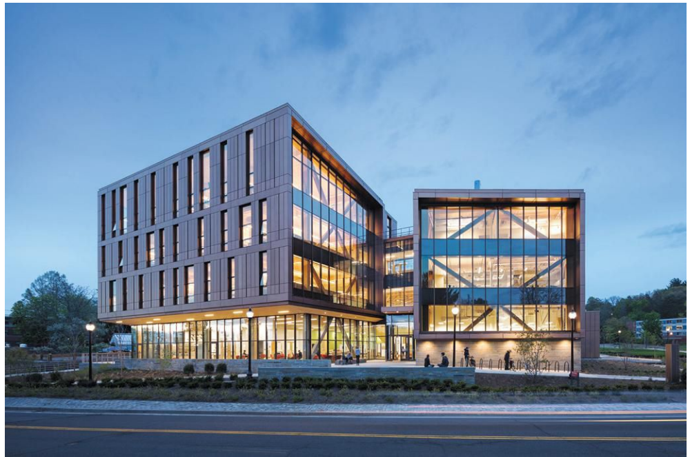
Designed as an innovative and inspiring building that visibly demonstrates the UMass Amherst's commitment to environmental sustainability, the John W. Olver Design Building uses a CLT structural system that significantly reduces its carbon footprint.
