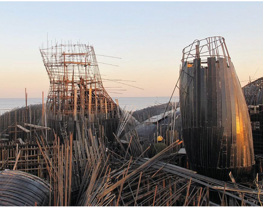
BY THE SEA The architects turned to local shipbuilders for the formwork (left and above). The inaugural exhibition explores the shifting relationship between humans and nature in light of China's last three decades of breakneck development (opposite).
