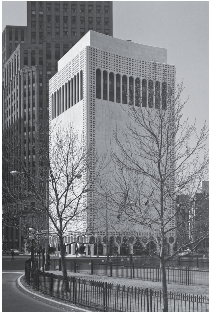
Banque Lambert, by Skidmore, Owings & Merrill (top). Gallery of Contemporary Art, by Edward Durrell Stone (bottom). Photos by Ezra Stoller, 1965 and 1964 respectively.
