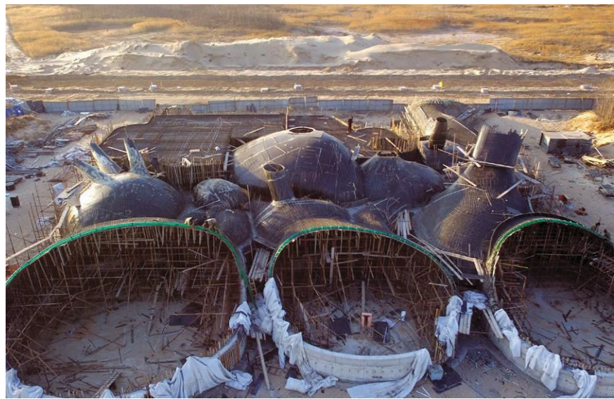
BY THE SEA The architects turned to local shipbuilders for the formwork (left and above). The inaugural exhibition explores the shifting relationship between humans and nature in light of China's last three decades of breakneck development (opposite).
