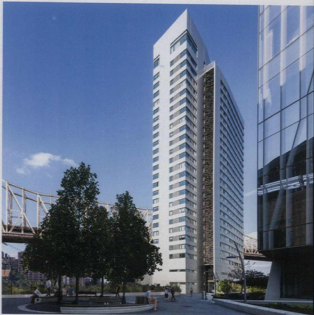
STANDING TALL The House (opposite), a 26-story residential tower, is slated to become the tallest and largest Passive House building in the world. Its superinsulated metal skin is expressed as a wrapper, with a vertical louvered reveal (above) that encloses mechanical equipment and extends from the entrance almost to the roof.
