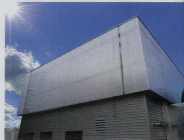
Cellular polycarbonate translucent glazing can provide daylighting facades for a variety of building types, including an integrated facade at Otterbein University (top) and Metro Tower III (bottom) which emulates the look of a frameless channel glass wall.
