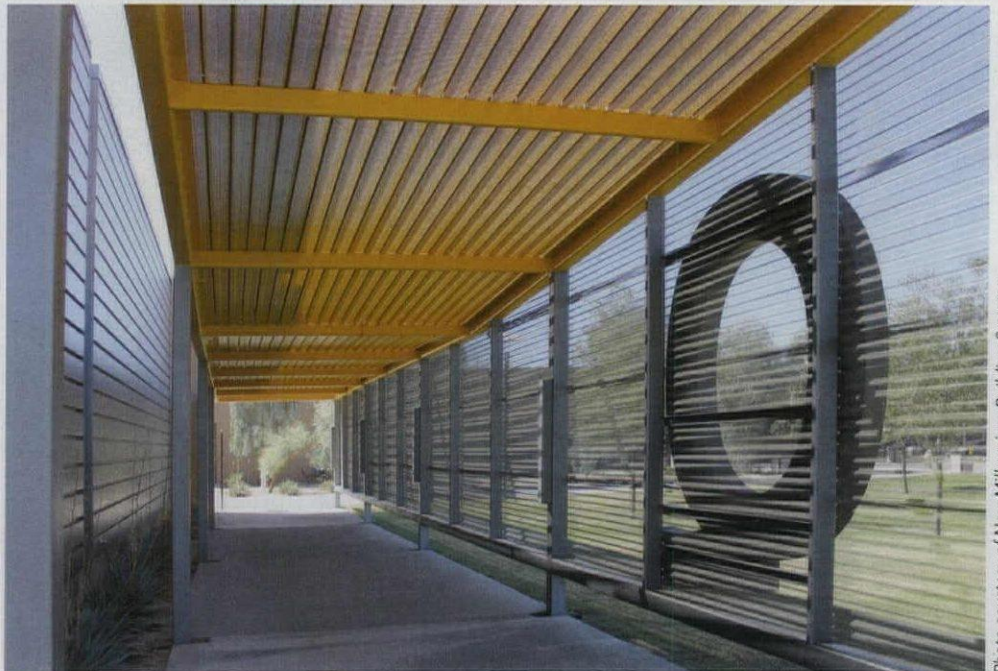
Pre-finished or stainless-steel deck can be used for a variety of building exterior applications, including vertical facades, horizontal canopies, or sunscreens and shades.
