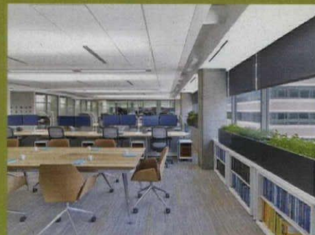
An automated shading system and PVC-free shade fabric helped the project to satisfy many of the credits that overlapped between the two green building systems.
