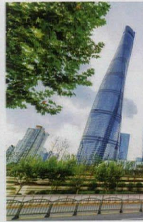
The Shanghai Tower, the world's second-tallest skyscraper, also featured an automated shading system and achieved a LEED Platinum rating for Core and Shell.
