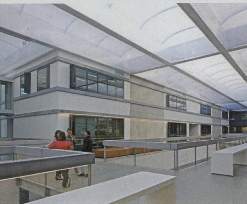
LIGHT FILLED A glass-roofed courtyard opens onto the main diagonal thoroughfare (this image). The oversailing ETFE roof offers daylit spaces throughout the large complex (below).
