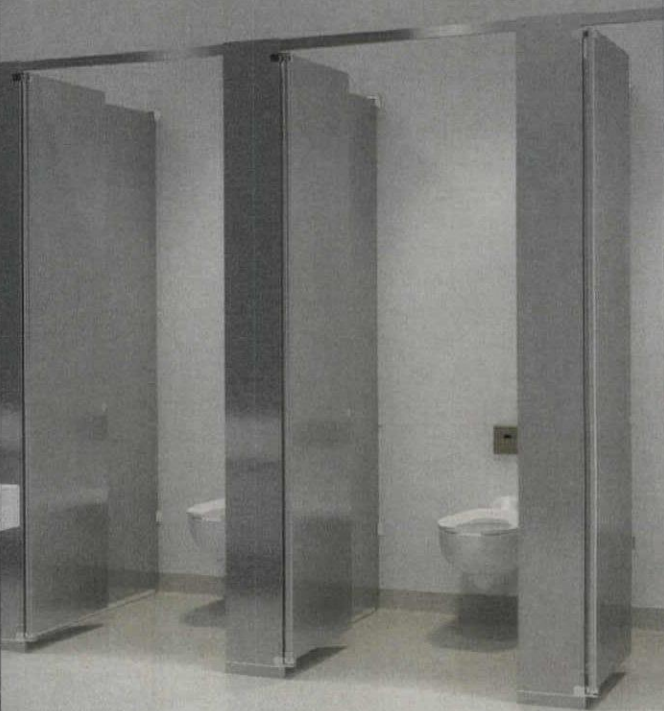
World-class commercial restroom design.
