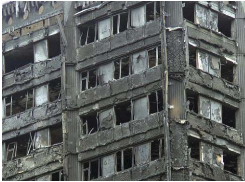
The Grenfell Tower disaster has led to combustibility testing in high-rise-building cladding across the United Kingdom.
