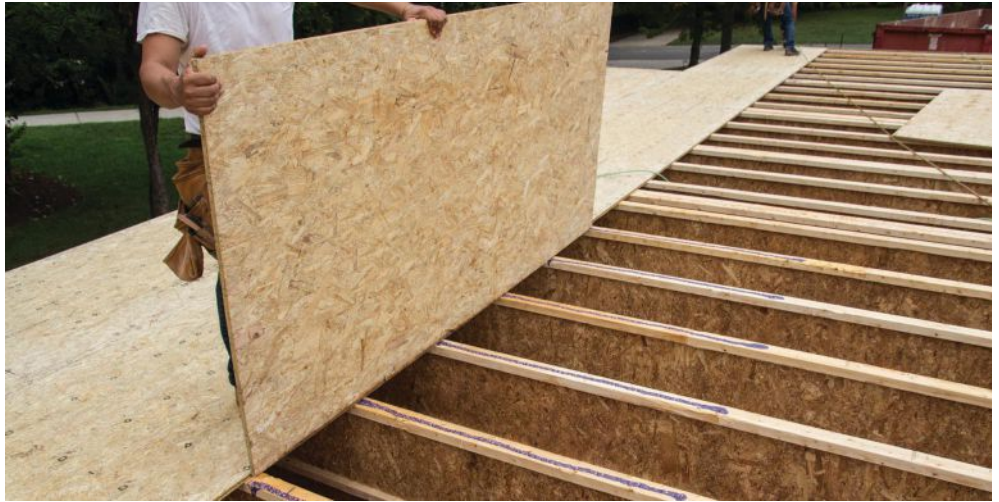
Structural floor framing elements, whether joists or trusses, need to be selected to work successfully with subfloor structural panels.
