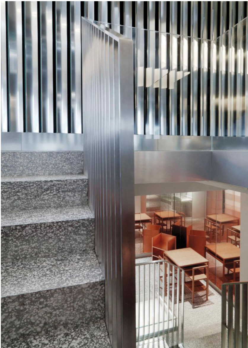
LEVEL OFF The staircase, sandwiched between the rotating billboard of the side walls, is a focal point (opposite). Its steps are formed from aluminum foam filled with resin that has the appearance of terrazzo (left). A wall of thick, sliding resin cases separates the office from the salon-style space on the lower level, furnished with Donald Judd tables and chairs (above).
