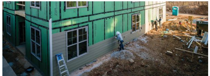
With a built-in water resistive barrier, ZIP System® sheathing and tape saves installation time by eliminating housewrap.
