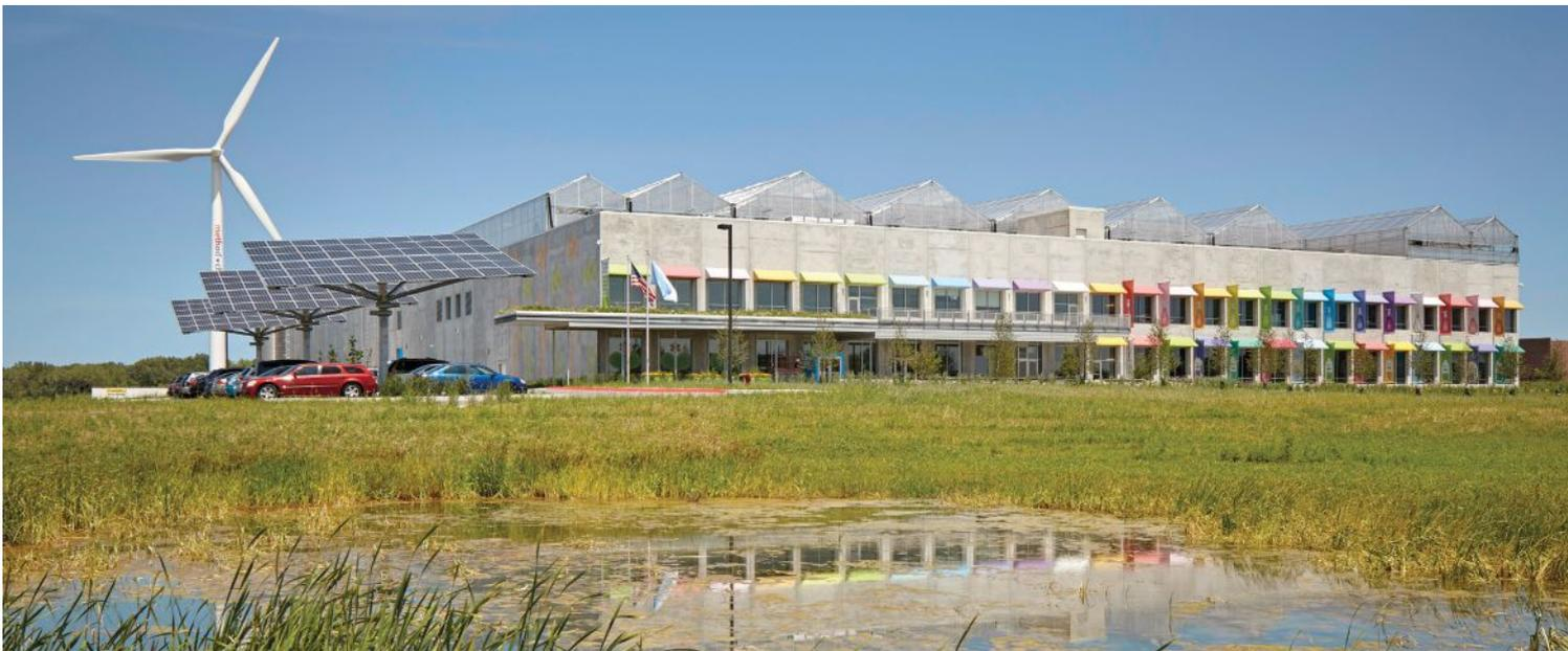
**INDUSTRIAL REVOLUTION** Architect William McDonough's Method cleaning products factory in Chicago (this page and opposite) has solar panels and wind turbines that satisfy about a third of its energy demands. The facility is constructed of materials vetted according to the C2C protocol, including paint, wall base, and adhesives.
