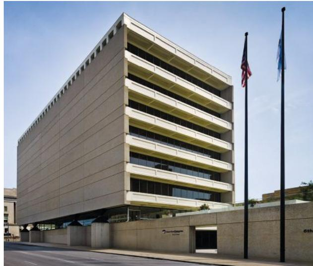
AEG’s headquarters, shown after the renovation, features poured-in-place walls supported on steel knuckles on the east and west (left), while its north and south (opposite) elevations are glazed. On the interior, BNIM recreated the effect of the original illuminated ceiling coffers. In addition to LEDs, sprinklers and other infrastructure are hidden above the replaced cylindrical ducts (below).
