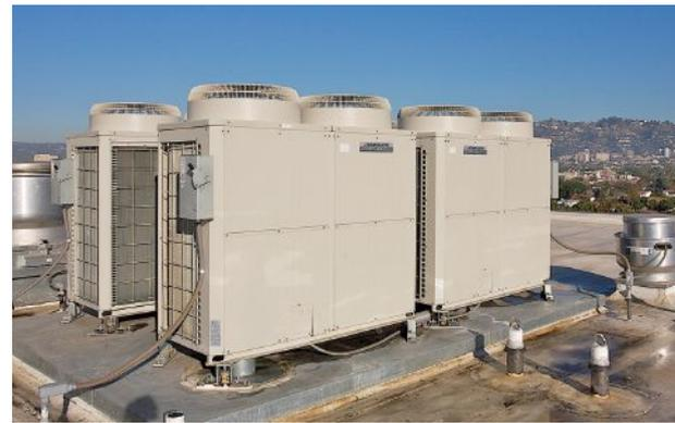
**Variable refrigerant flow (VRF) zoning systems use centrally cooled or heated refrigerant run to individually zoned spaces based on the demand for space cooling or heating.**
